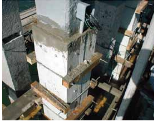
Lifejacket filled with concrete
