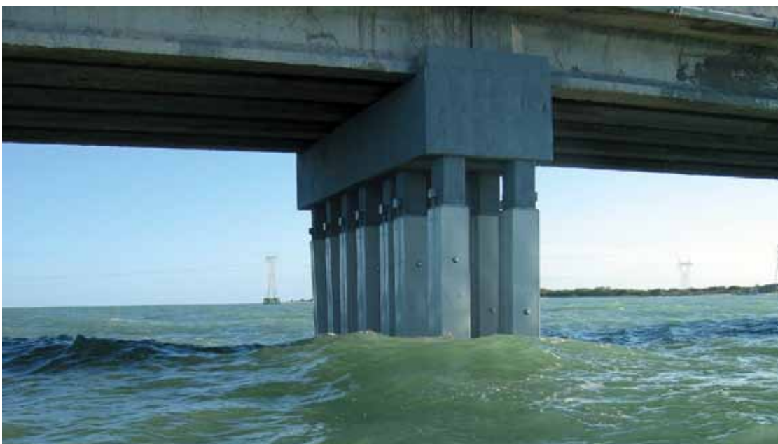
Completed installation of Lifejacket® and metalized zinc cathodic protection systems
