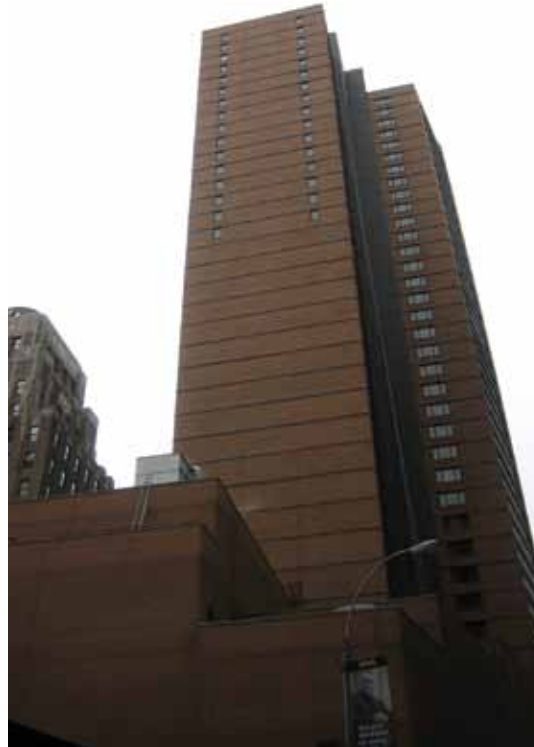
East elevation and shear wall elevation after completion of repairs
