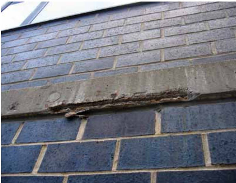
Exposed concrete slab edges as observed during engineering survey
