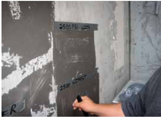
Concrete shear wall coating surface preparation and bond test prototypes
