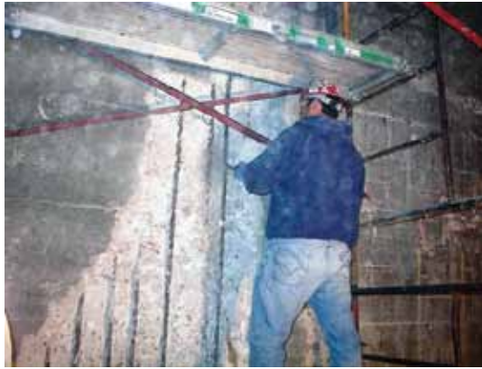
Surface preparation with chipping hammer on foundation walls
