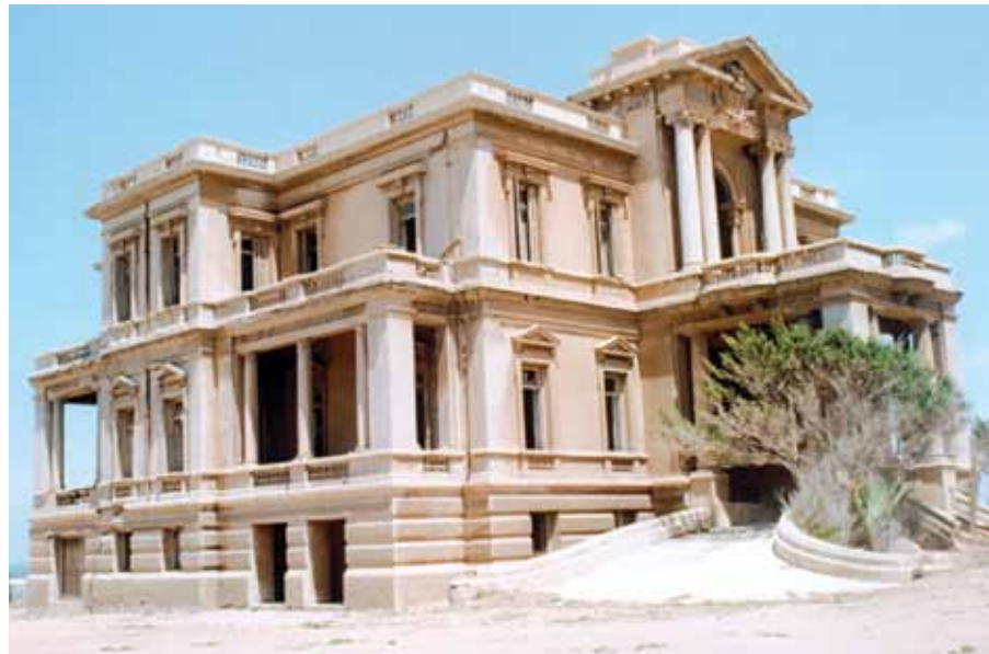
Fig. 1(a): The palace, showing perspective of the east and the south façades
