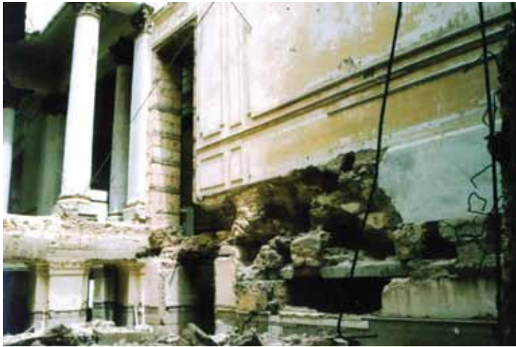
Fig. 2: Photographs showing basement roof and top roof removed harshly
