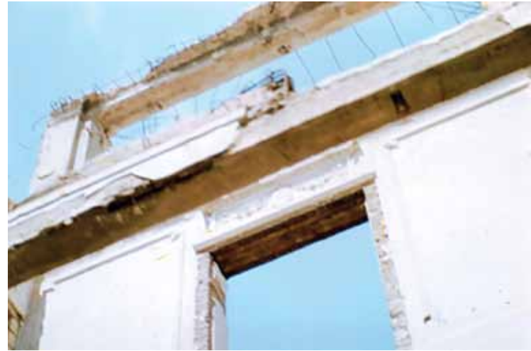
Fig. 2: Photographs showing basement roof and top roof removed harshly
