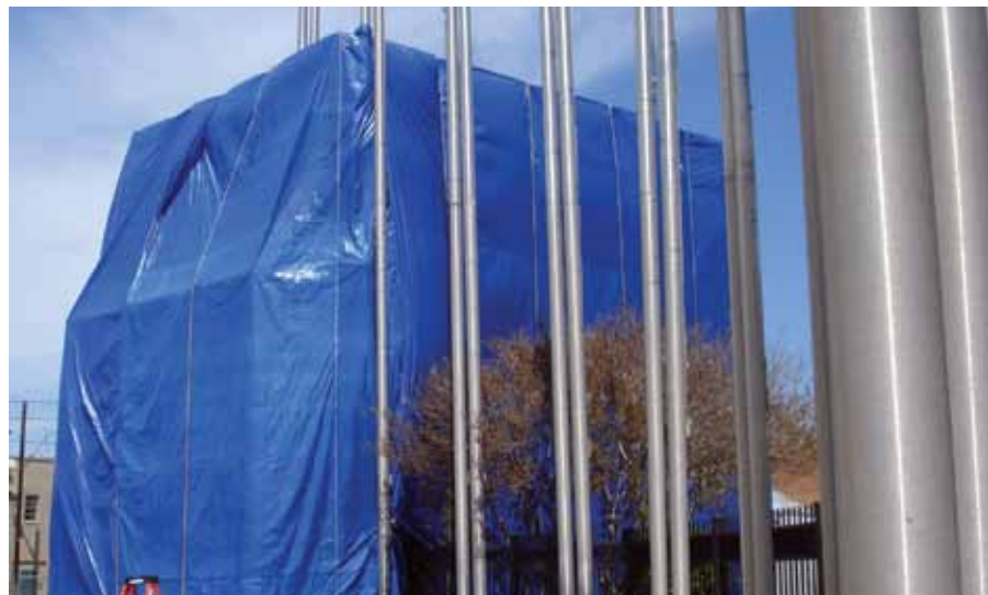
Ticket booth with tarp covering for containment of lead-paint removal
