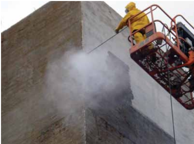
Parry Avenue Central Tower being cleaned
