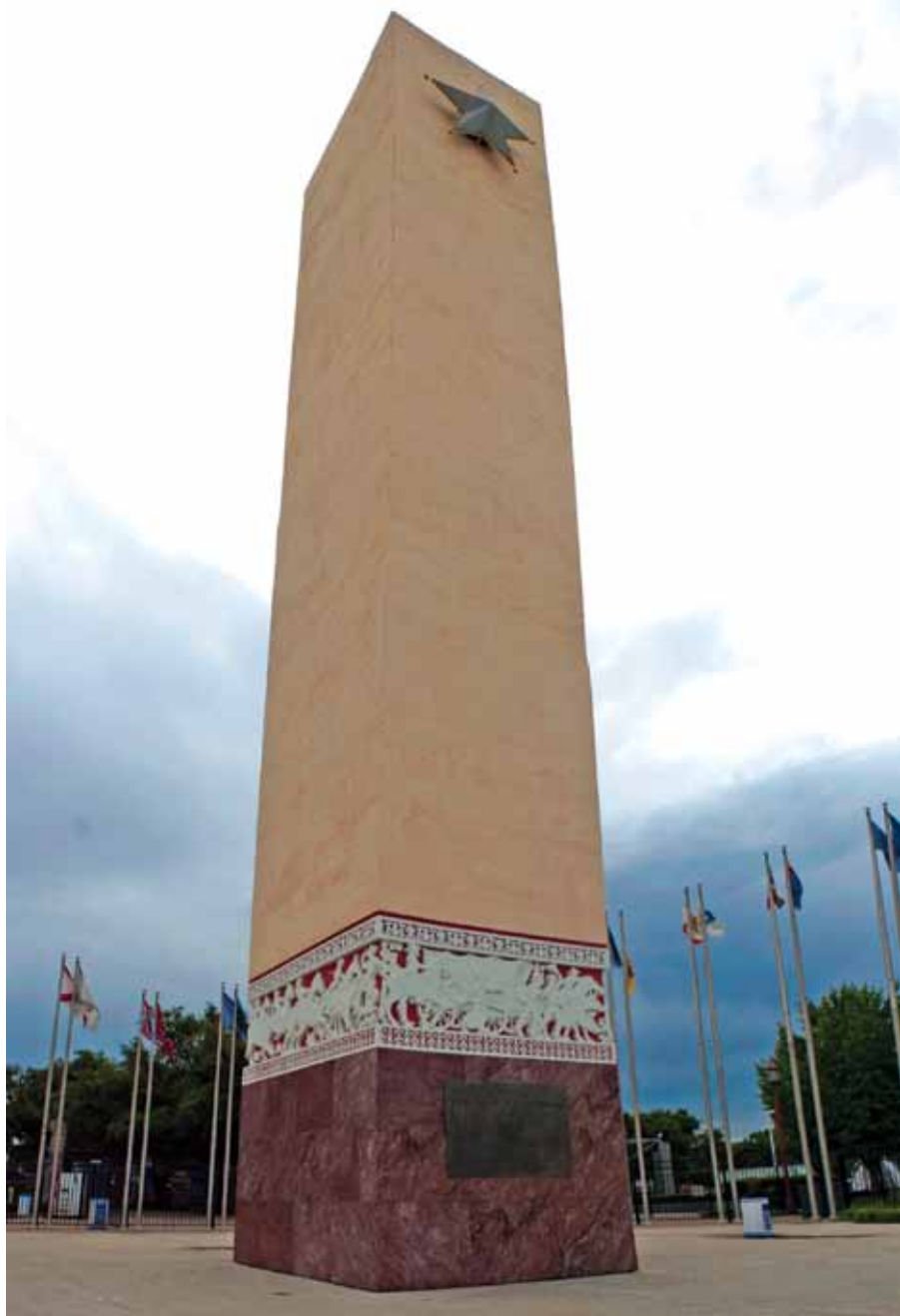
Central Tower after restoration
