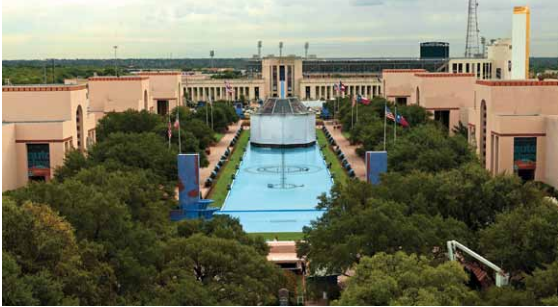
Completed Esplanade fountain and reflecting pool
