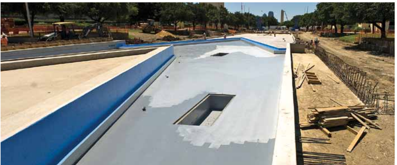
Waterproofing the Esplanade fountain and reflecting pool
