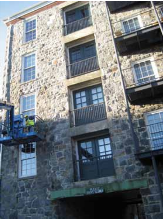
Nearly 2400 sills and lintels were repaired
