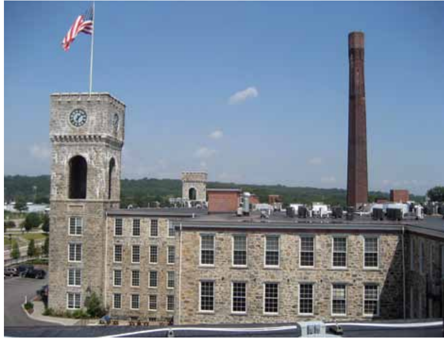
The waterproofing project was finished ahead of schedule and on budget
