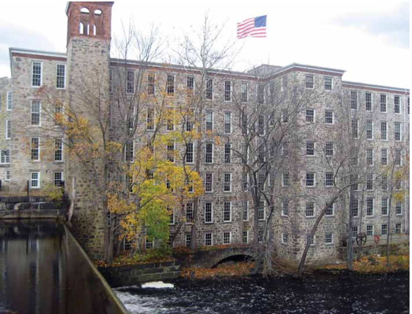
The riverfront location and waterfall posed a waterproofing challenge
