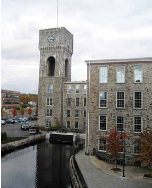
Canal dam head section received extensive reconstruction to stave off canal head pressure from lower apartment units
