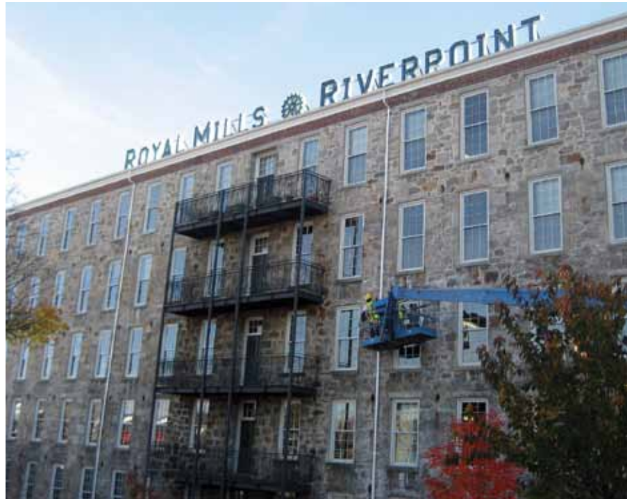
Extensive stone veneer repair work was completed
