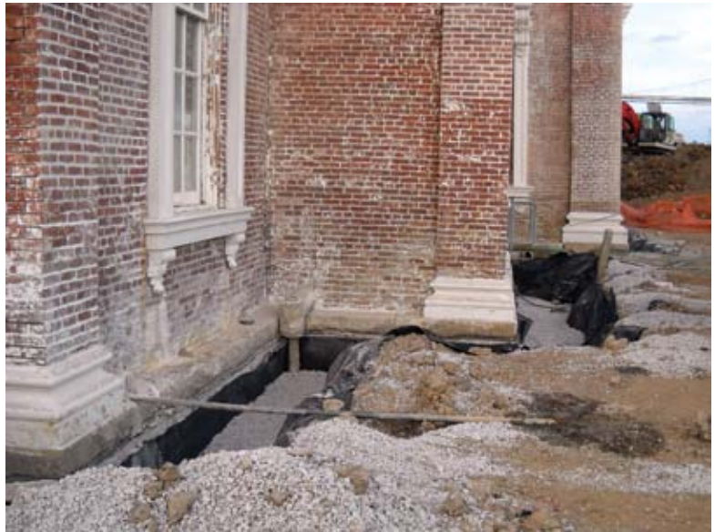
West elevation waterproofing excavation and north elevation waterproofing installation
