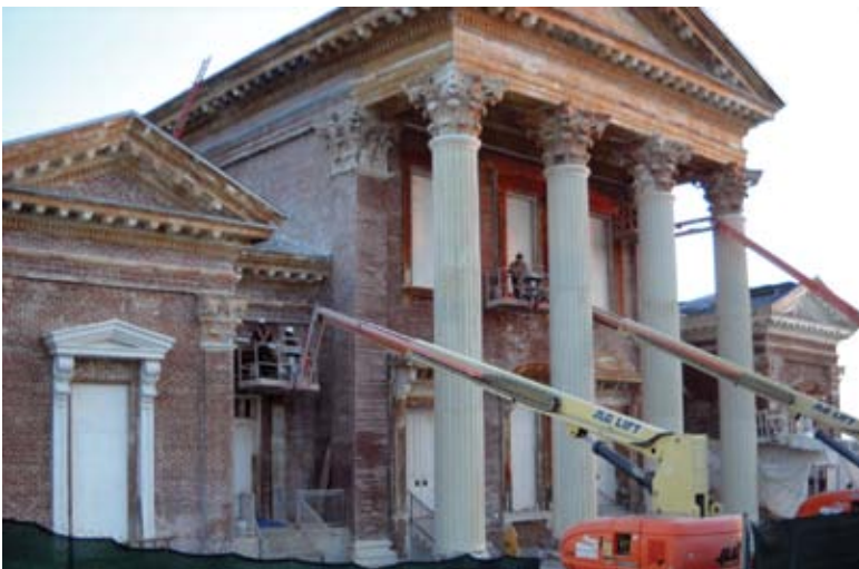
Project during restoration
