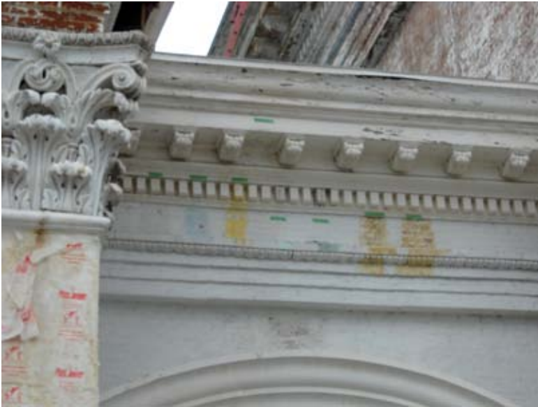
Different product mockups were tested to determine the most effective coating removal product
