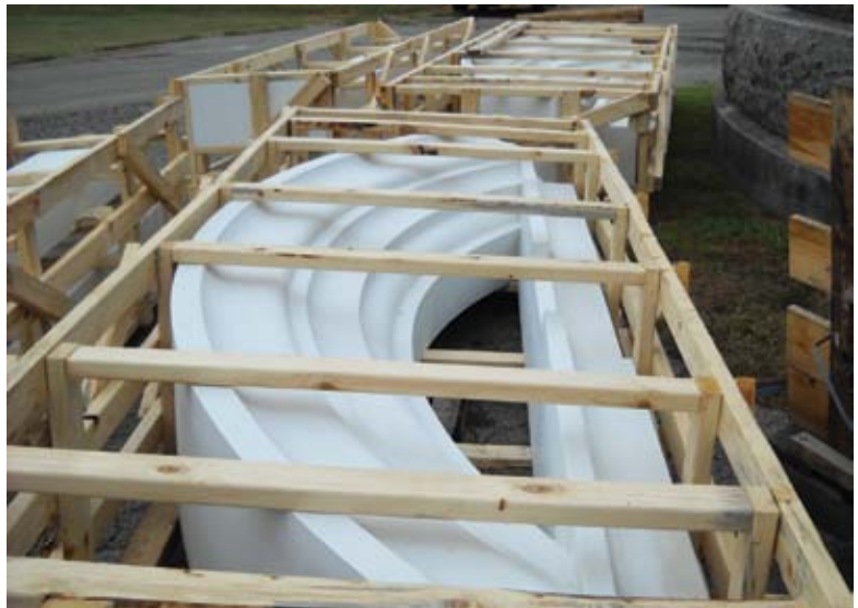
GFRC piece replicated to match the existing cast iron door surrounds
