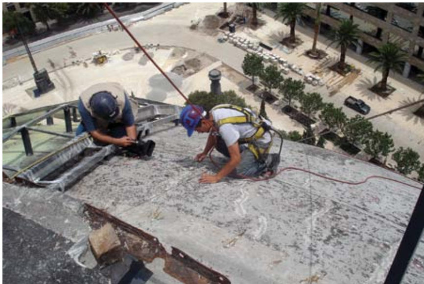
Crack injection
