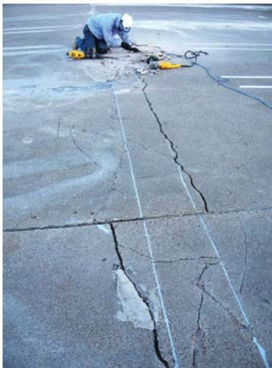
Fig. 2: Crack and concrete spall repair
