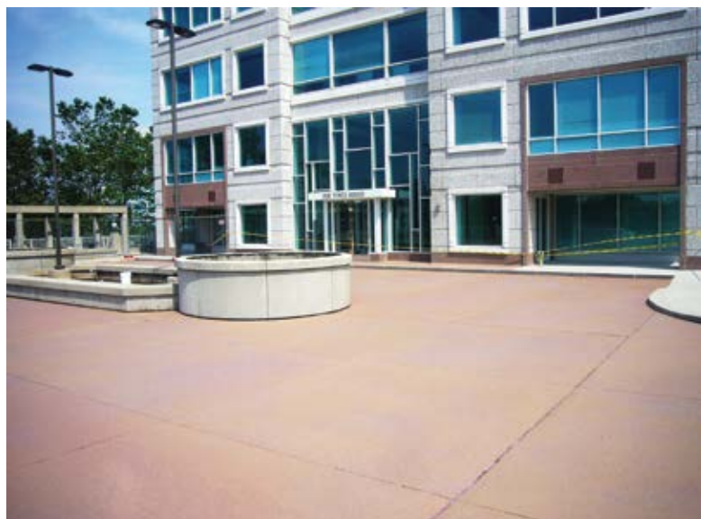
Fig. 1: Waterproofing membrane applied to pedestrian plaza
