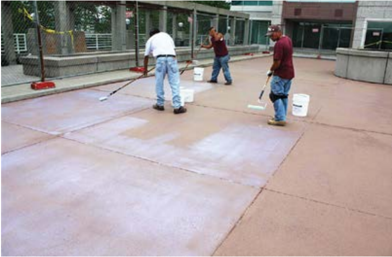
Fig. 4: Primer application during polyurethane system installation
