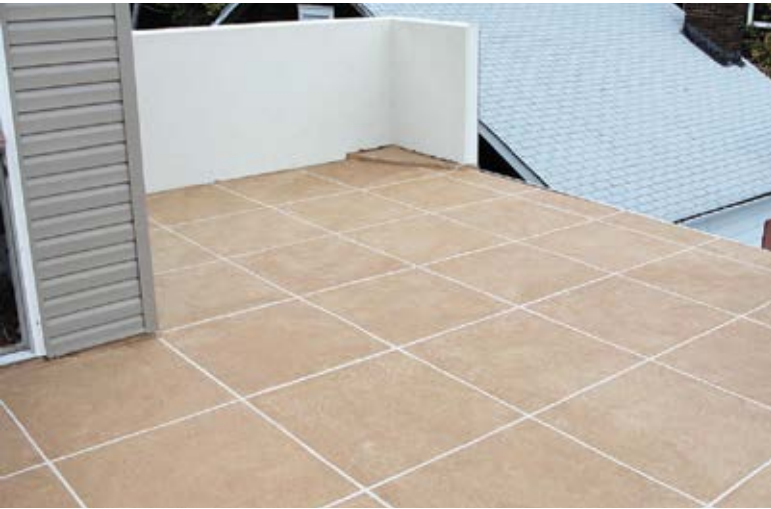
Fig. 5: Waterproofing system installation at deck
