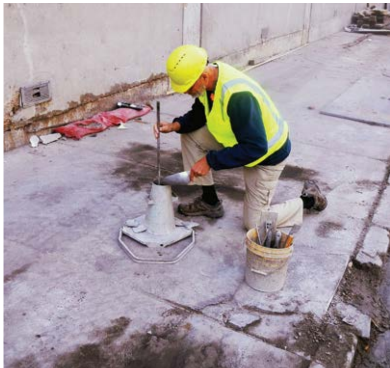
Fig. 1: Testing for slump
