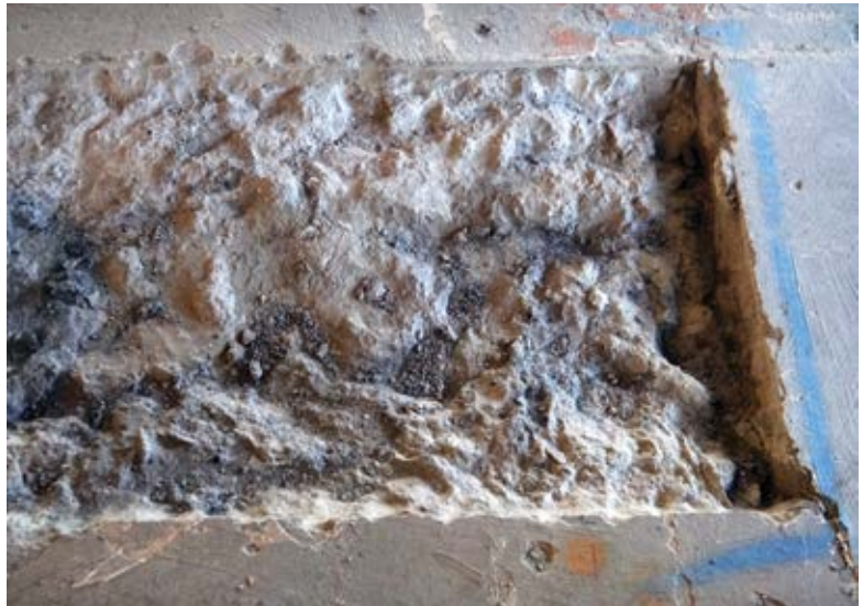
Fig. 8: Selectively demolished partial-depth repair area at top of slab
