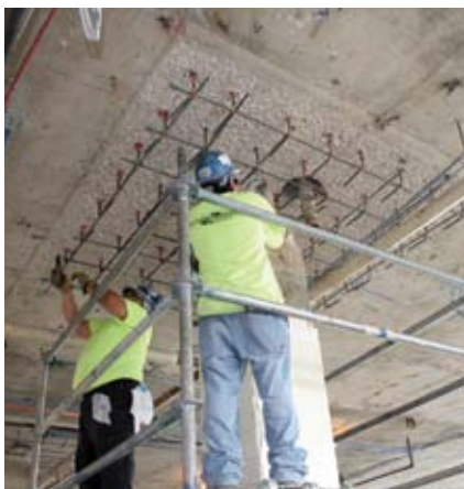
Installing reinforcement for concrete drop-panel enlargements
