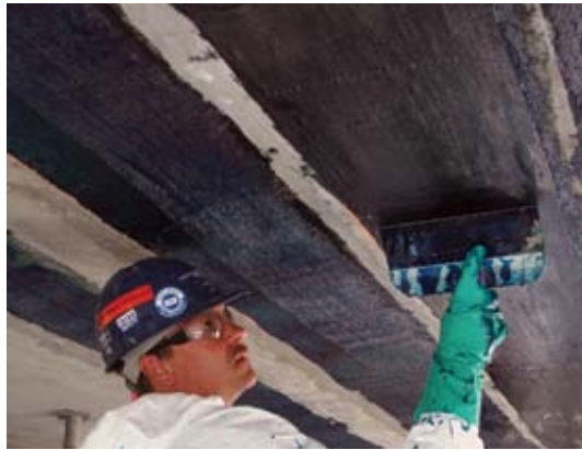
Installation of CFRP sheets on the underside of the slab
