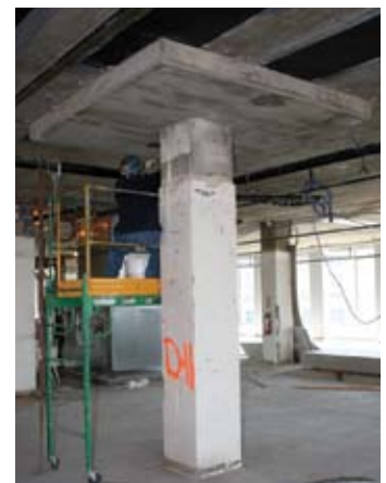
Completed concrete drop-panel enlargements
