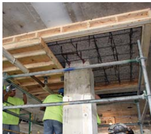
Installing forming for concrete drop-panel enlargements
