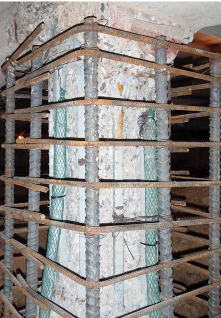
Fig. 8: Galvanic encasement protects and strengthens severely damaged columns
