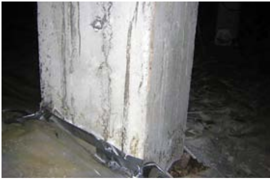
Fig. 4: Column with no damage (green condition)
