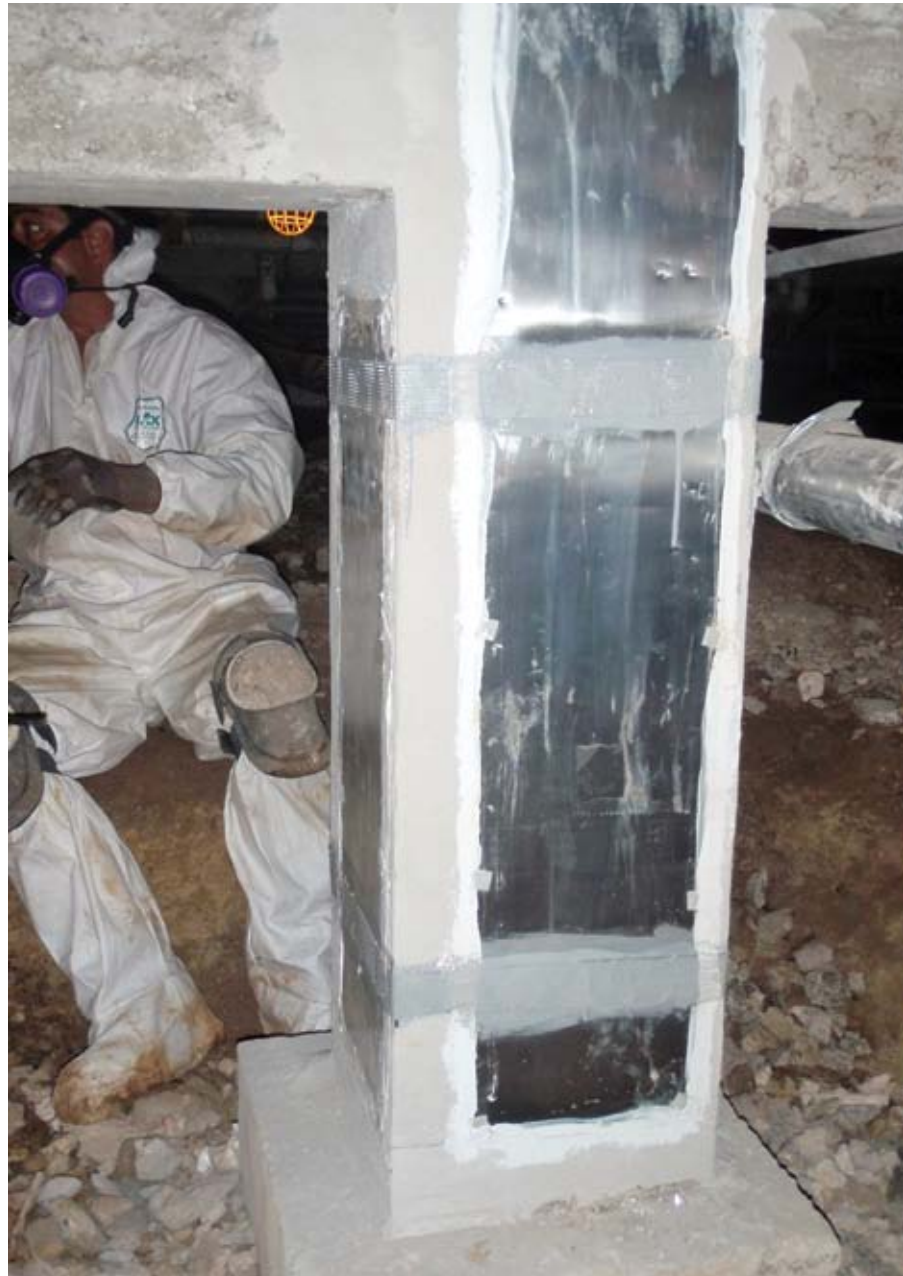
Fig. 9: Surface applied zinc sheet anodes prior to final coating
