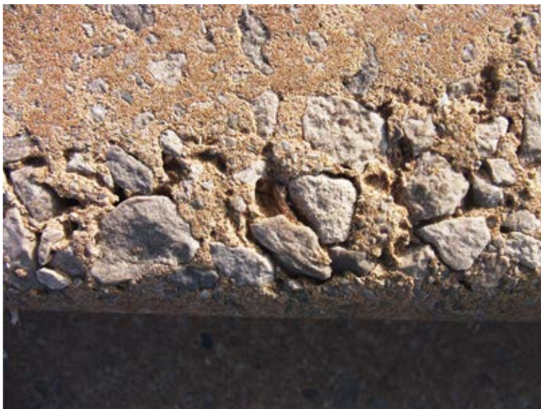
Fig. 7: Nose of the step of the unit shown in Fig. 6 after 5 years' exposure
