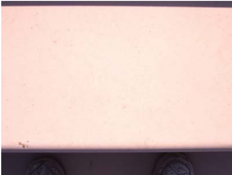
Fig. 6: Newly placed concrete tested in this research
