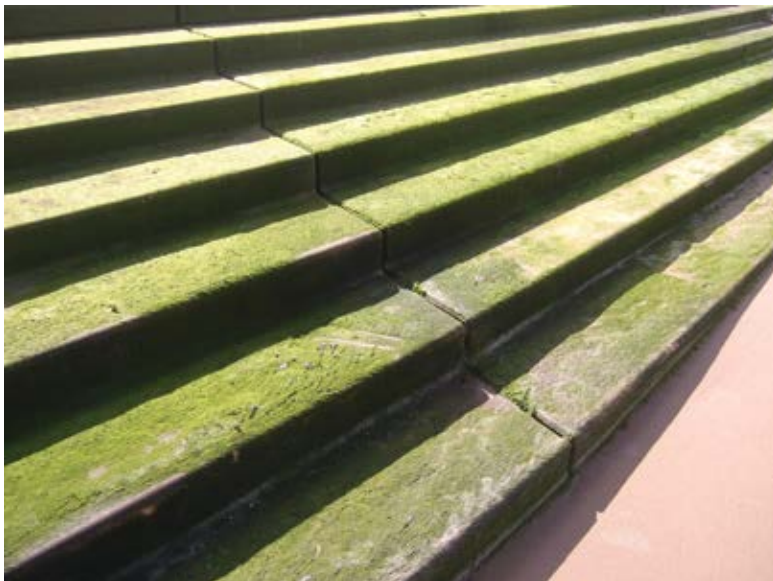
Fig. 2: Revetment armor steps colonized with algae
