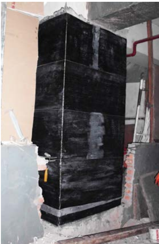
Fig. 3: Columns strengthened with carbon wrap
