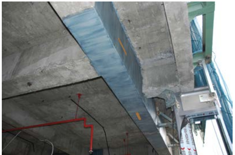
Fig. 4: Reinforcement of beam with CFRP
