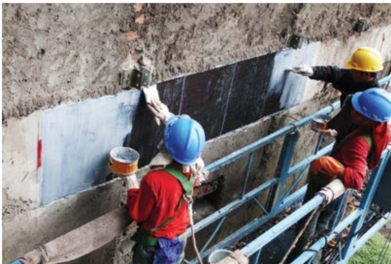
Fig. 7: Application of adhesive to previous CFRP layer
