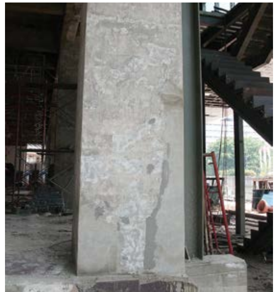
Fig. 9: Patched column section
