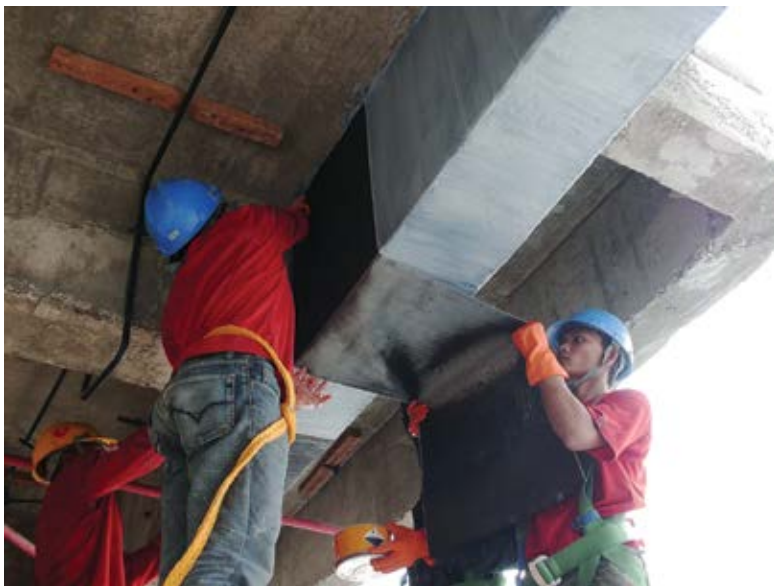
Fig. 6: CFRP being placed on adhesive
