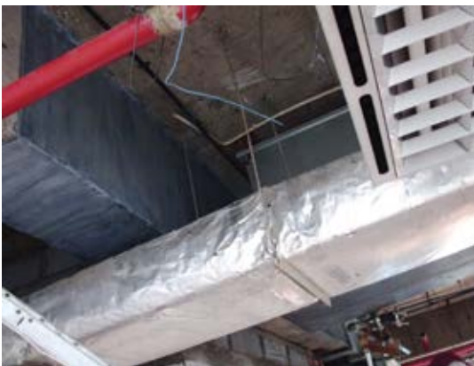
Fig. 12: CFRP installed around existing obstacles
