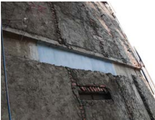
Fig. 11: Beam strengthened without removing wall
