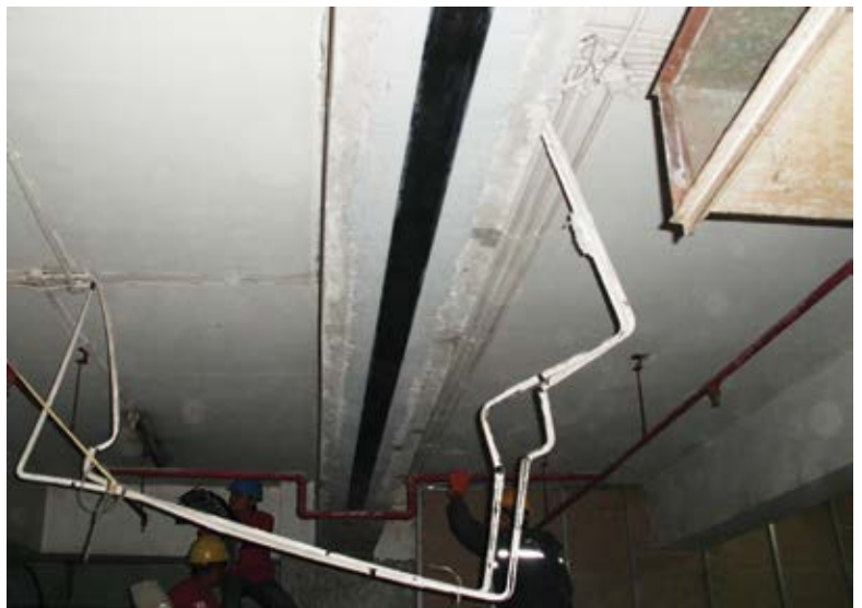
Fig. 5: Reinforcement of beam with carbon plate
