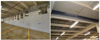
(c) Precast double tee beams and precast (d) Steel frame with concrete on metal deck light walls
