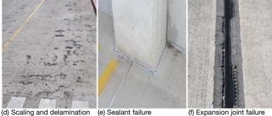
Fig. 3: Common types of deterioration in parking structures
