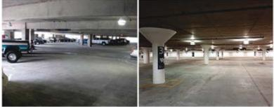
(a) Cast-in-place long span post-tensioned (b) Cast-in-place flat slab post-tensioned
