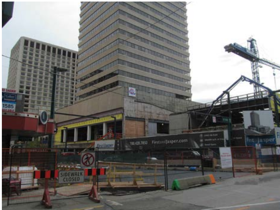
Fig. 1: Overall view of project site during construction
