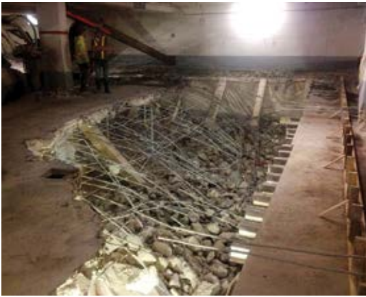
Fig. 6: Slab demolition in progress
