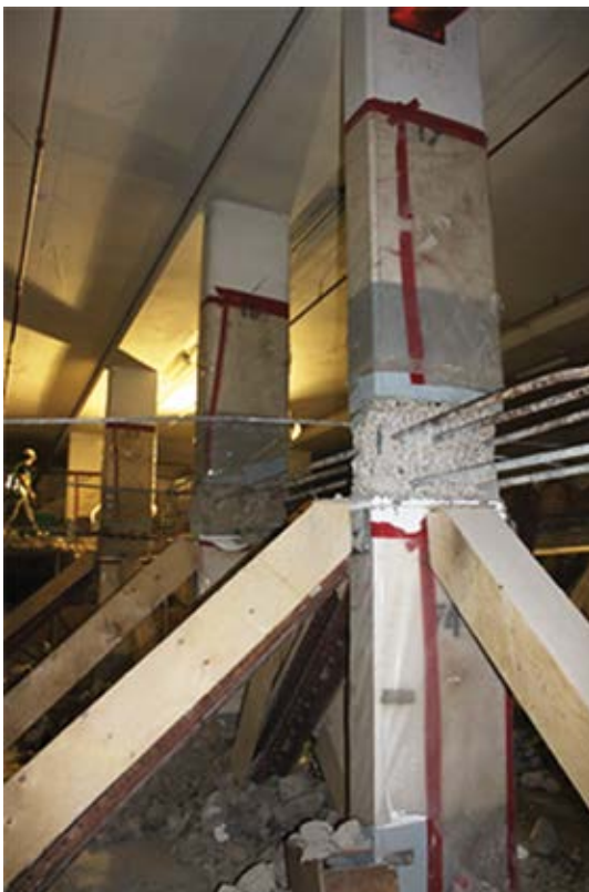
Fig. 4: Interior concrete columns braced to maintain load-carrying capacity
