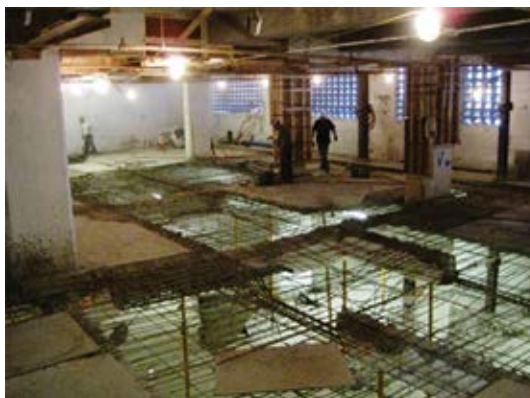
Fig. 9: Demolition in preparation for full-depth slab and beam replacement
