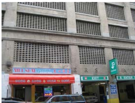
Fig. 5: Shoppers Garage, May 2008, showing concrete masonry screens and storefronts (Photo courtesy of CCE)
