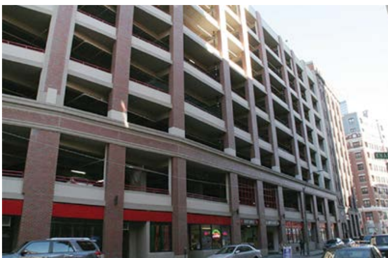
Fig. 8: Beach Street façade after renovation in late 2013
