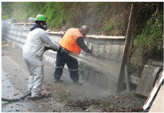
Fig. 1: Dry-mix shotcrete being installed on a retaining wall project
