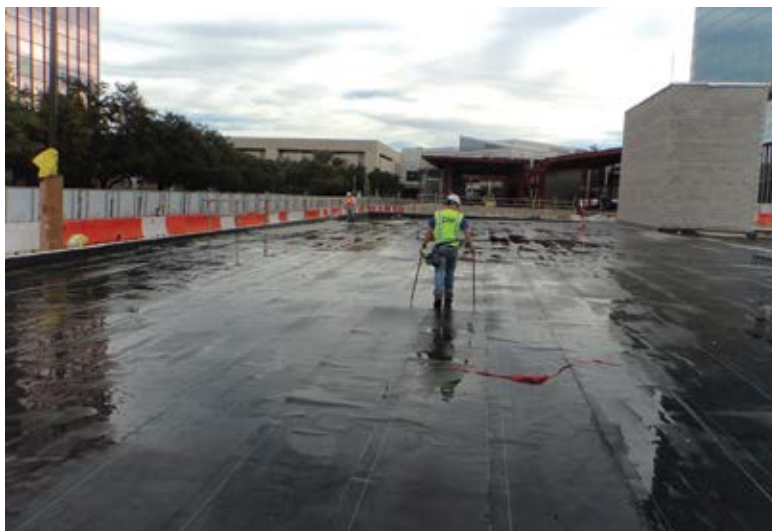
Fig. 2: LVELD testing in progress
