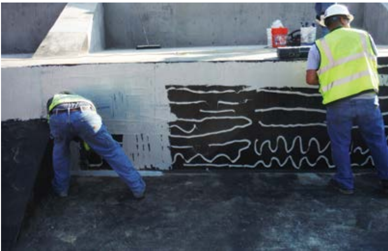
Fig. 5: Retroactive sealant application to repair pinholes
