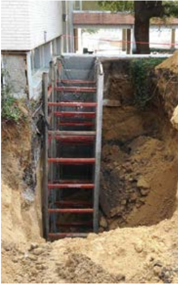
Fig. 7: Trench box in the narrow excavation site
