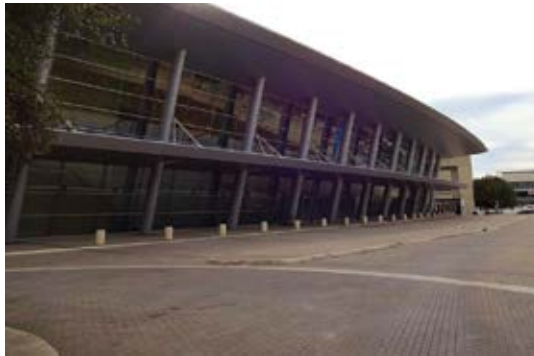
Fig. 9: The area of Ceremonial Drive under which the convention center's storm drain system resides
