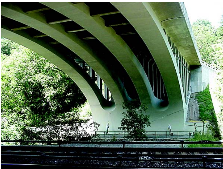
Access to the arches was restricted by a commuter railroad and river
