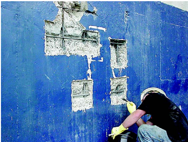
Cleaning spalled areas prior to repair
