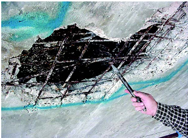
Typical spall on underside of thin shell
