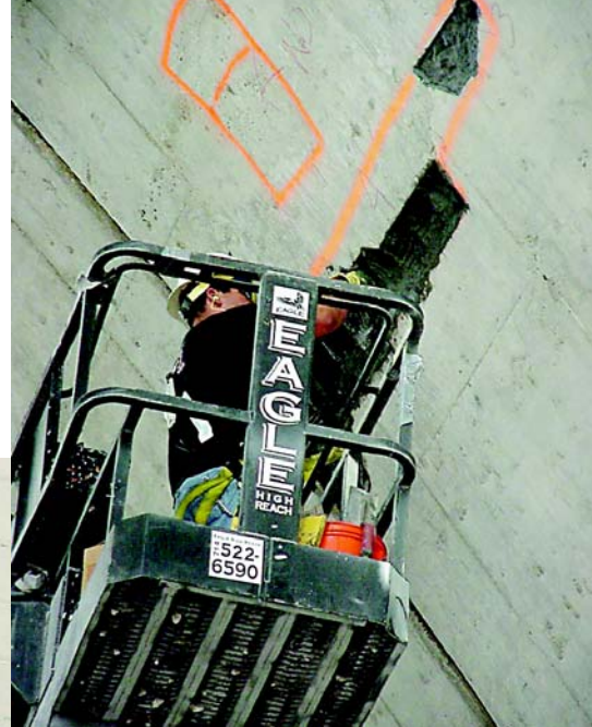
Repairing spalls
