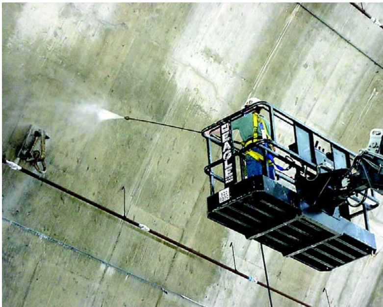
Surface preparation by hydroblasting
