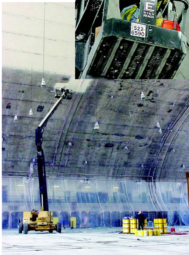
Applying coating to exposed concrete surfaces
