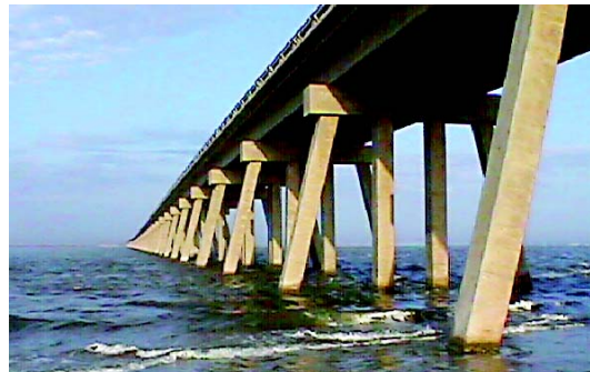
Figure 2: San Luis Pass Bridge, Galveston, Texas
