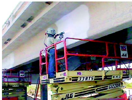
Figure 3: Arc spray application of aluminum-zinc-indium (Al-Zn-In) anode
