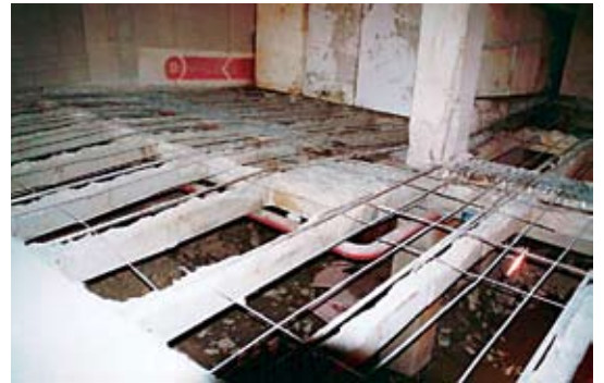
Full-depth concrete removal
