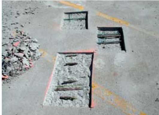
Removal of deteriorated concrete
