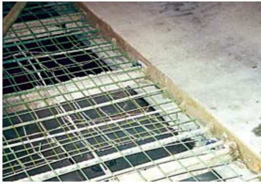
New reinforcing steel on pan and joist system
