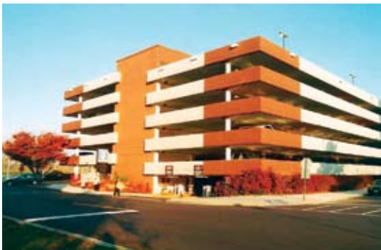
Completed view of exterior of parking deck
