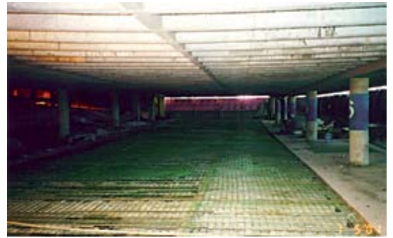
Full-depth slab replacement
