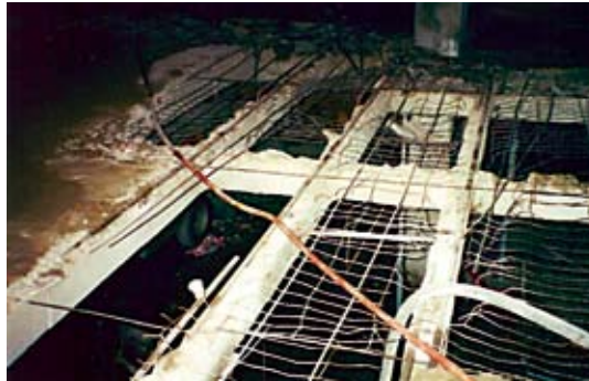
Concrete removal using hydrodemolition
