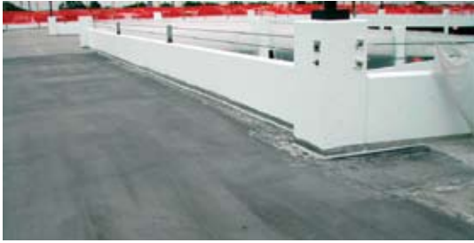
New deck coating
