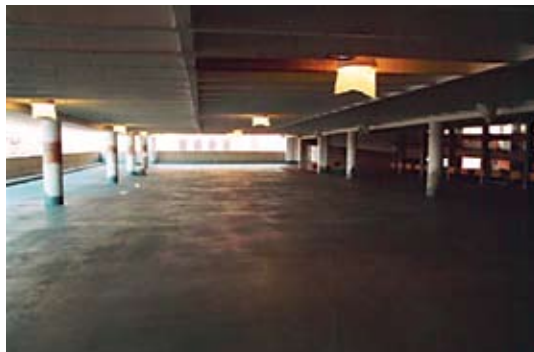
Completed view of interior of parking deck
