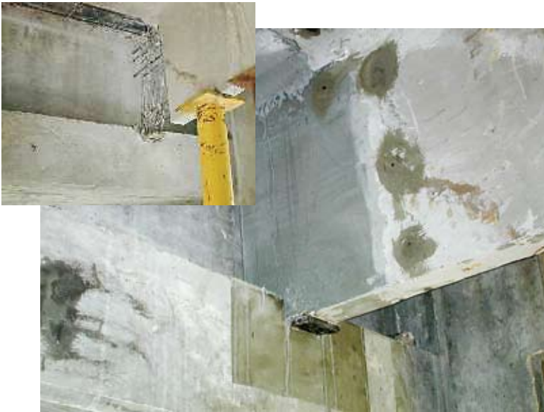
Fig. 4 (top inset): Beam repair in progress
