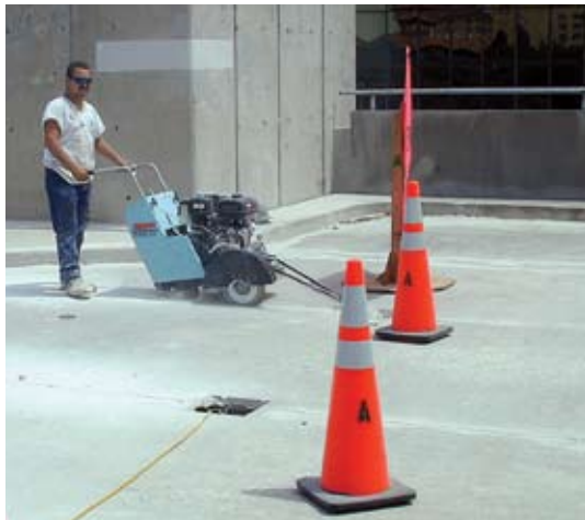
Fig. 6: Concrete cutting and removal at top level
