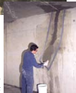
Applying slurry to concrete crack
