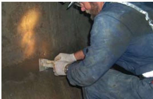
Packing crack with dry pack
