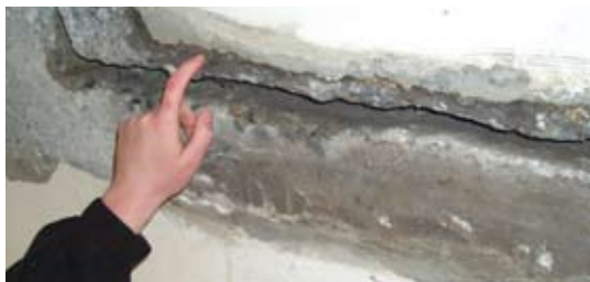
Chipped-out crack ready for dry pack
