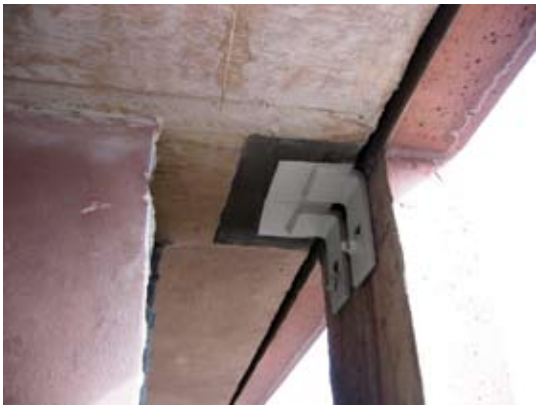
Fig. 5: Repaired precast column connection
