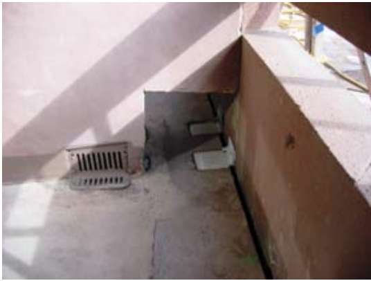
Fig. 4: Repaired precast wall connection on slab
