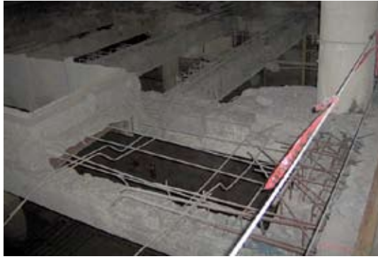
Floor perforations being built
