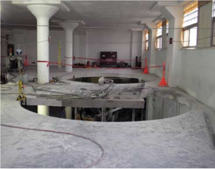
New floor with perforations ready for equipment
