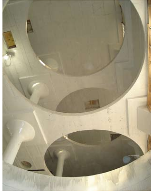
Looking up through bin holes in new floor slabs
