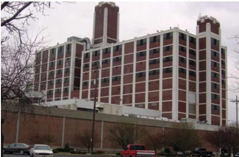
Exterior of 10-story plant
