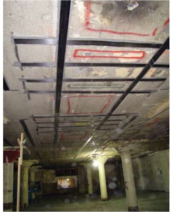
CFRP installed in ceiling
