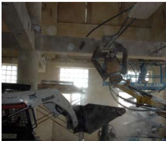
Demolition of interior beams
