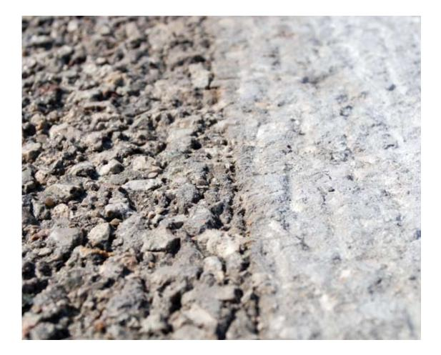
process. HSS uses truck-mounted equipment with a 2 ft (0.6 m) wide scarifying head, capable of carrying 4000 gal. (15,140 L) of water and generating 36,000 psi (248 MPa) of water pressure. The truck is connected to a vacuum system allowing for a neat and efficient scarifying operation. Production rates averaged 30,000 ft<sup>2</sup> (2787 m<sup>2</sup>) per shift.
