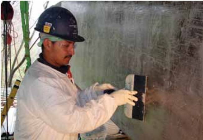
Smoothing of surface using putty filler for holes and cracks
