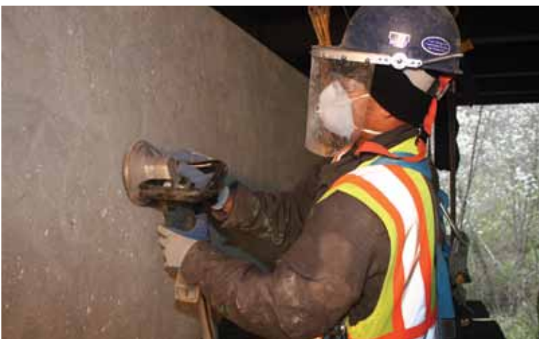
Surface preparation of concrete
