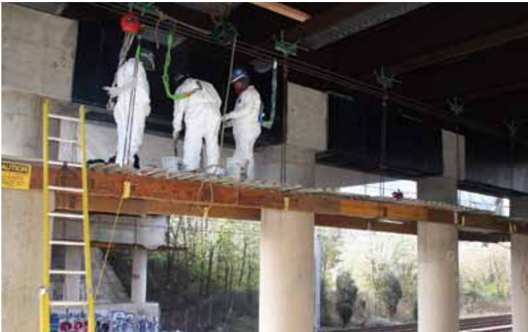
Elevated work deck allowed for access around entire work area
