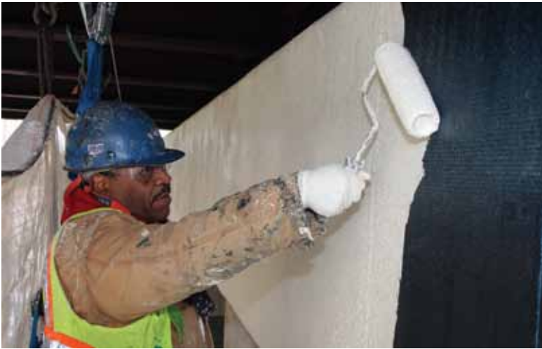
Application of topcoat for aesthetics and improved durability
