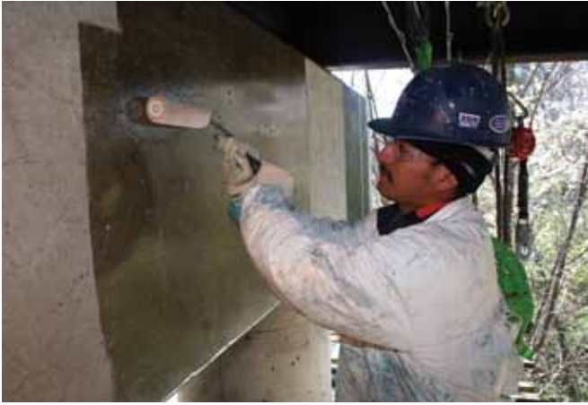
Application of surface primer
