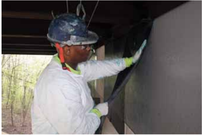
Saturated carbon fiber sheets are placed onto the primed surface
