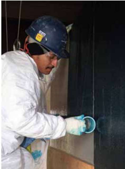
Saturated carbon fiber sheets are rolled onto the structure
