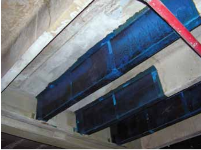
Fig. 4: Carbon fiber mesh installation
