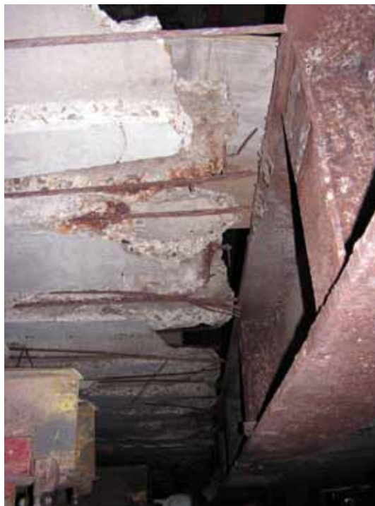
Fig. 2: Double-tee end demolition (from below)
