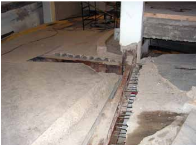
Fig. 6: Steel beam replacement/repair
