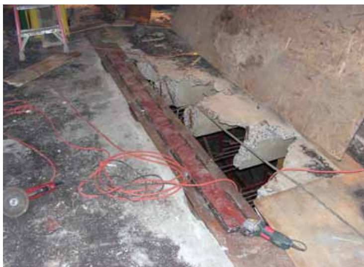
Fig. 3: Double-tee end demolition (from above)
