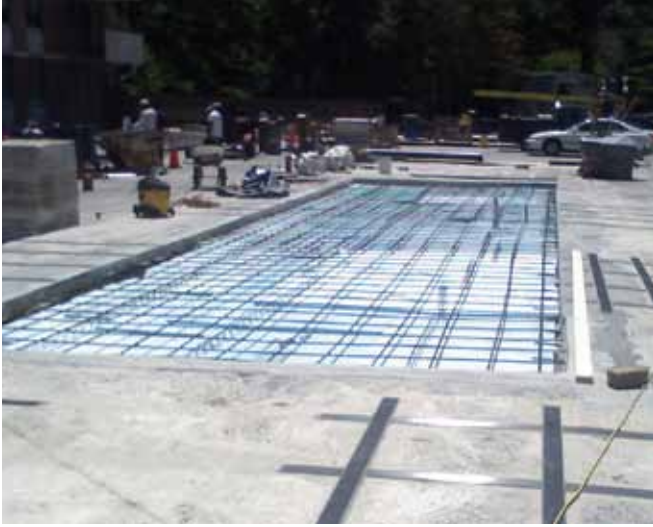
Existing fountain areas were filled in
