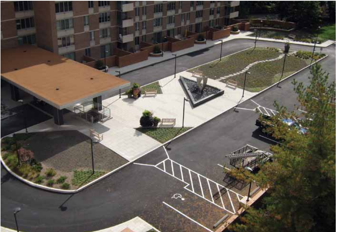
Plaza and landscaping after the rehabilitation was complete
