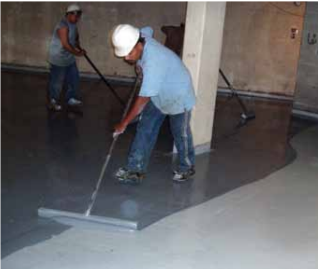
A vehicular traffic-bearing membrane coating was applied to the upper-level garage
