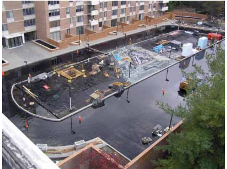
The entire plaza was water tested for 24 hours
