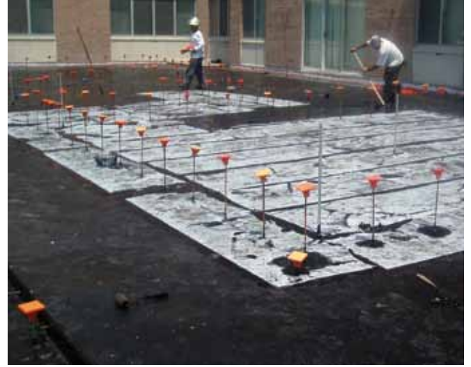
A hot-applied rubberized asphalt membrane was installed on the plaza deck
