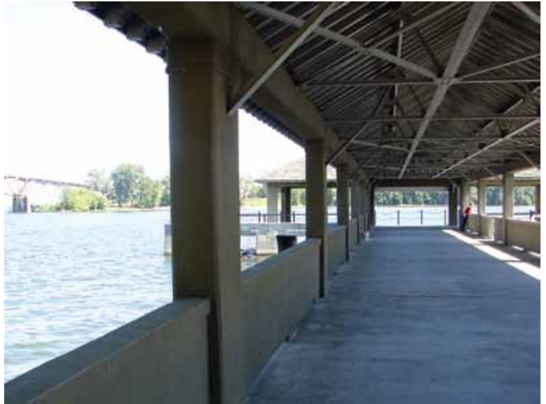
The finished pier, completed on time and on budget
