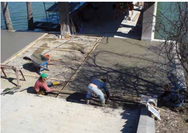
Repairing the approach slab with new concrete
