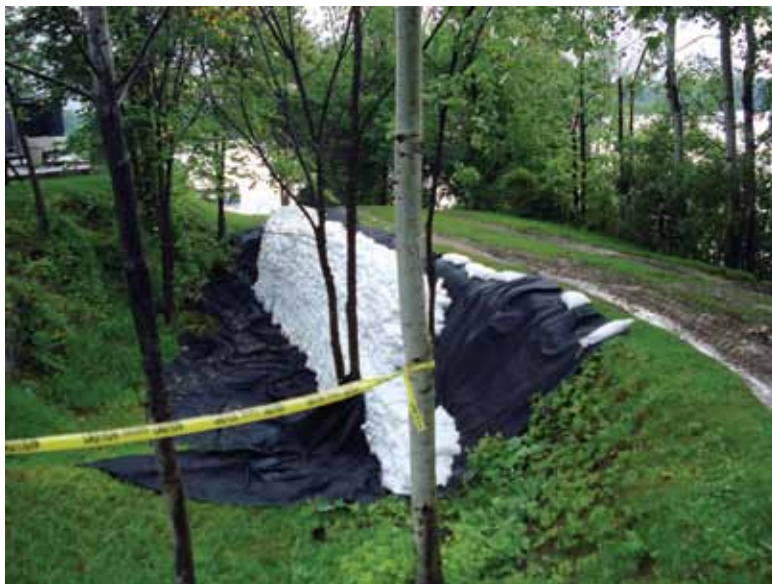
Stone and earth walls of the historic fort redoubts being protected by sandbags
