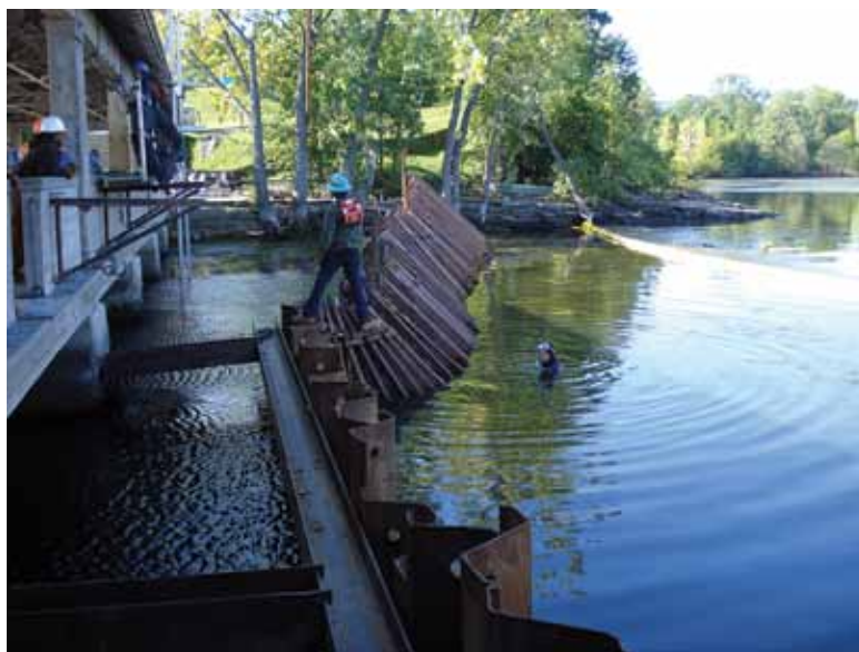
Erection of portable fabric cofferdam in shallow areas
