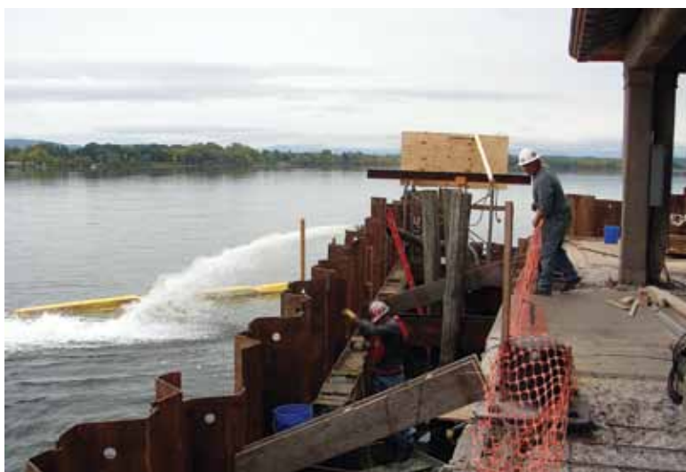
Dewatering of the cofferdam
