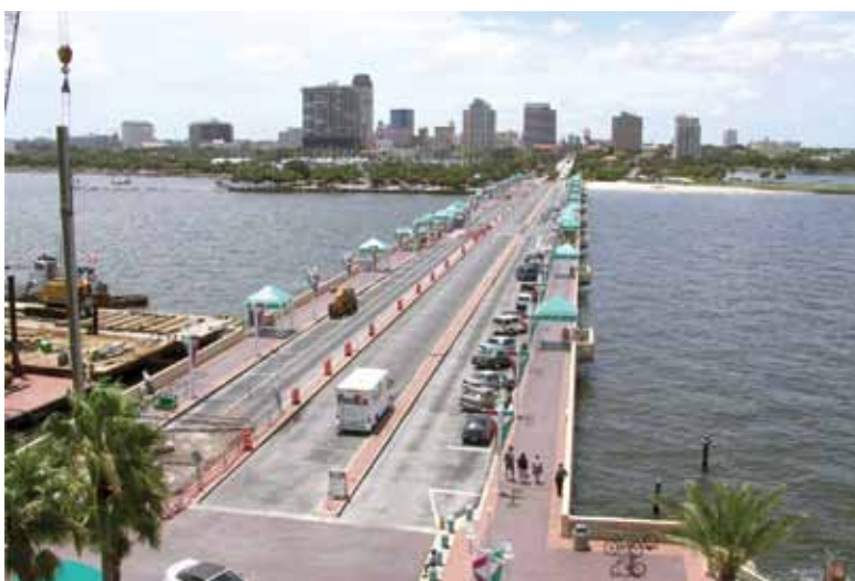
Approach to pier
