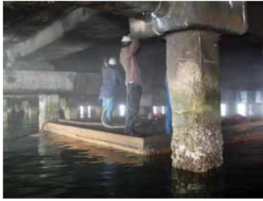
Floating work area under pier
