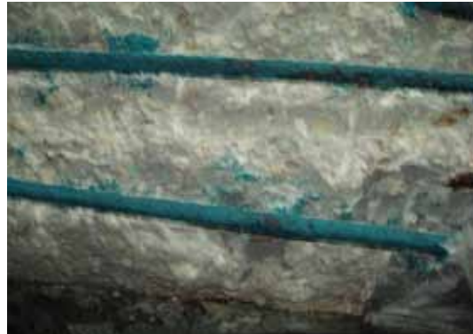
Newly exposed reinforcing steel protected with a water-based epoxy-cementitious coating
