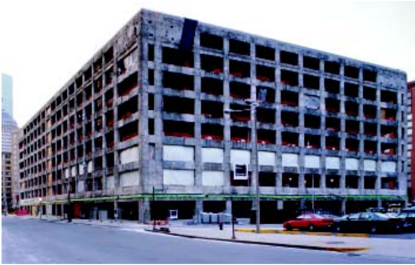
Facade from Stuart St. & Broadway Corner (during)
