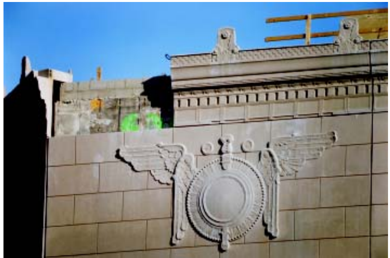
Facade detail (during)
