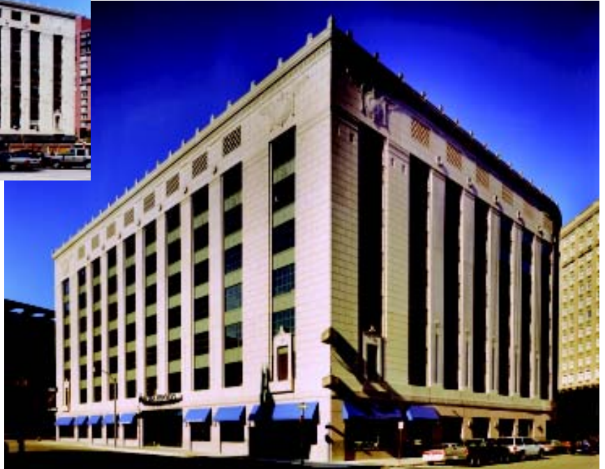
Facade from Stuart St. & Broadway Corner (after)
