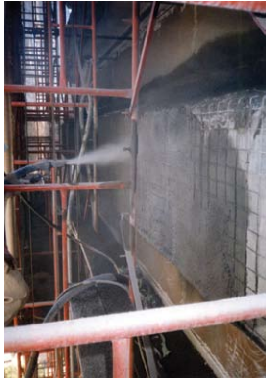
Shotcrete in progress
