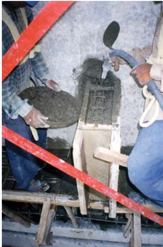
Bracket concreting and compacting using a needle vibrator
