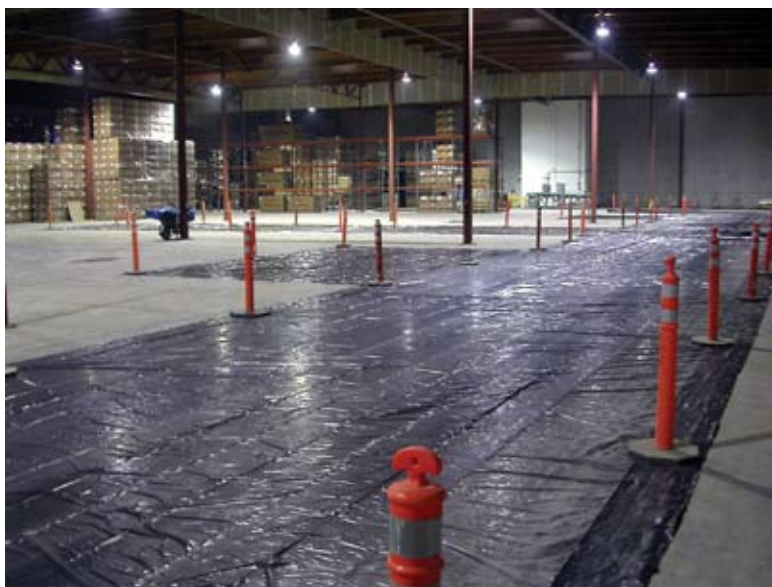
Floor slab curing
