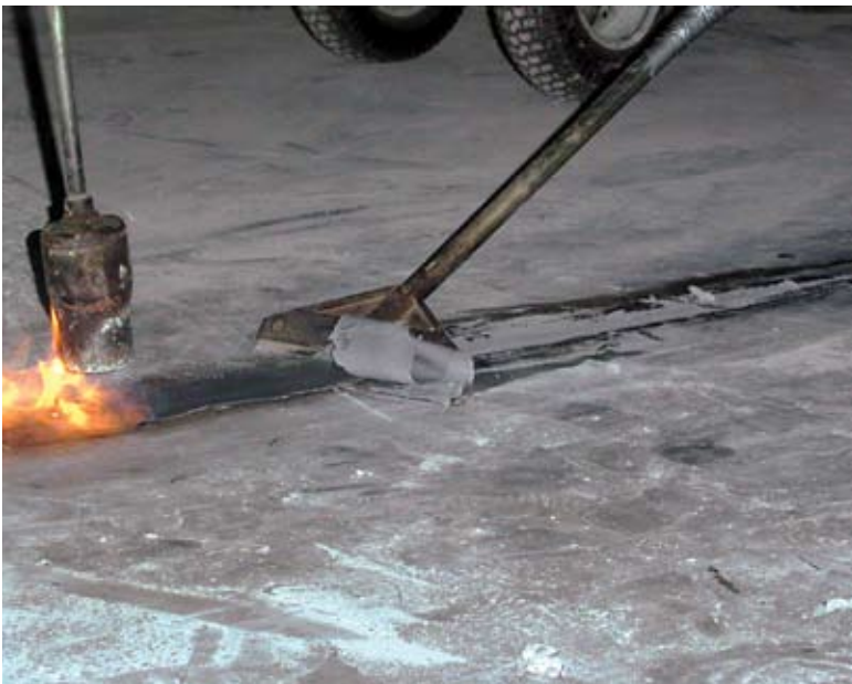
Cutting of semi-rigid epoxy filler at control joint
