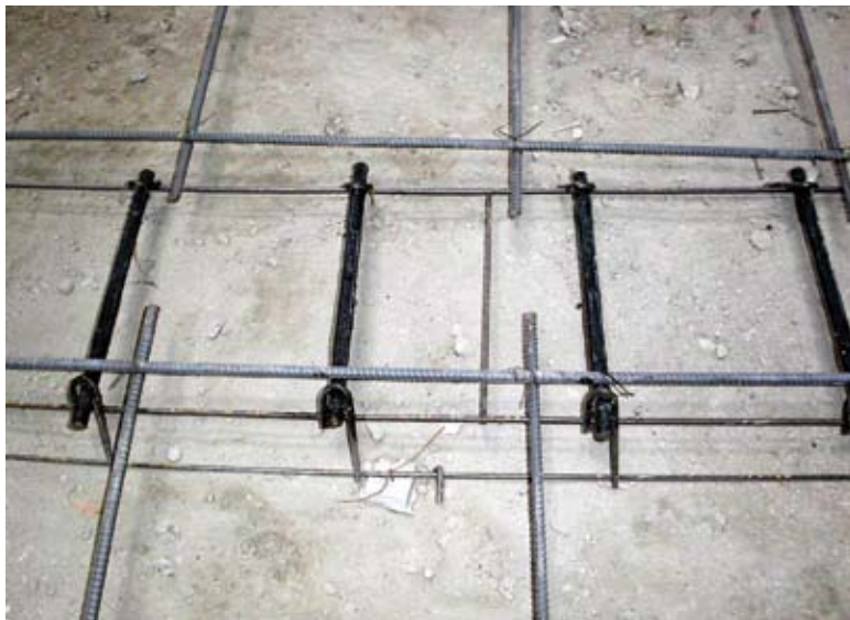
Greased round dowels at new-to-new slab joint
