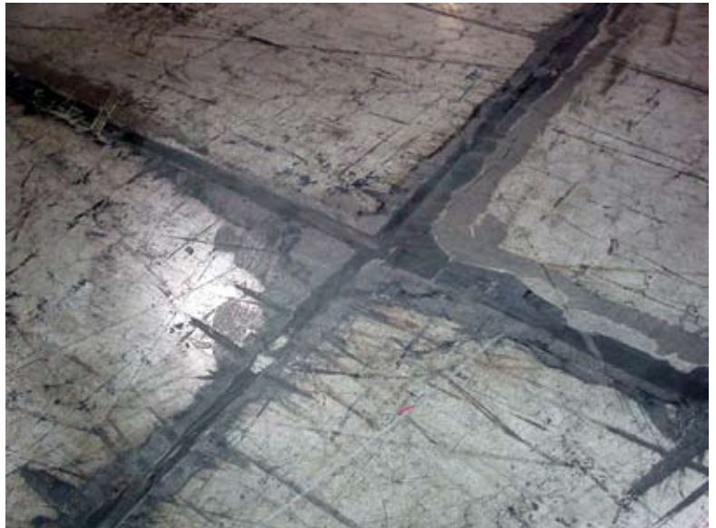
Epoxy joint and spall repair in existing slab after one year
