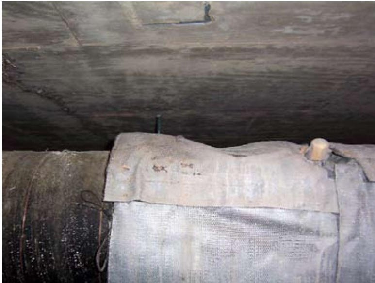
Fig. 7: Soffit of tunnel after restoration (compare to Fig. 3)
