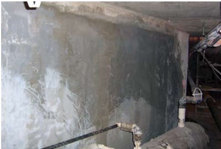
Fig. 8: Northwest diagonal wall after restoration (compare to Fig. 4)
