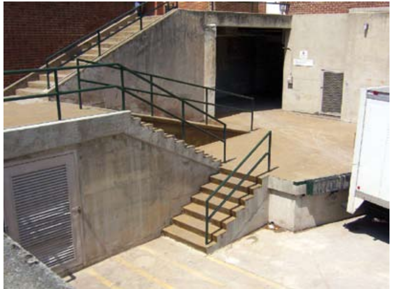
Fig. 10: Overview of finished project after restoration
