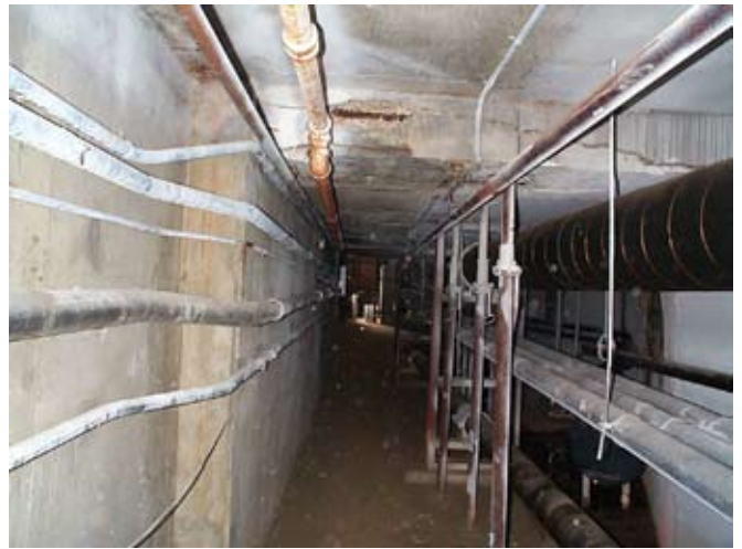
Fig. 6: Spalling and reinforcing steel corrosion in the concrete beam over the tunnel
