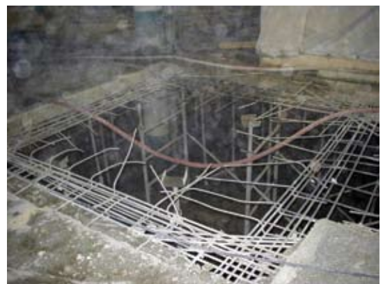
Full-depth repair at a crane opening
