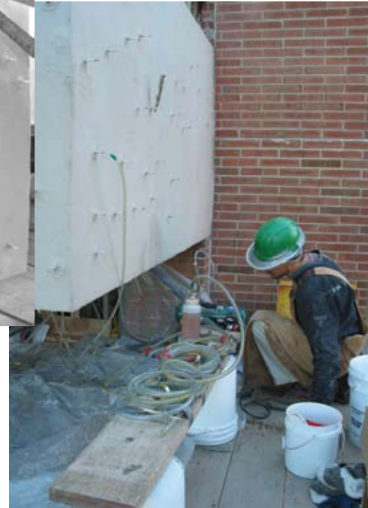
Vacuum injection of resin
