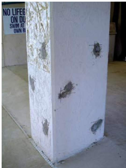
Anodes installed into column on staggered grid pattern
