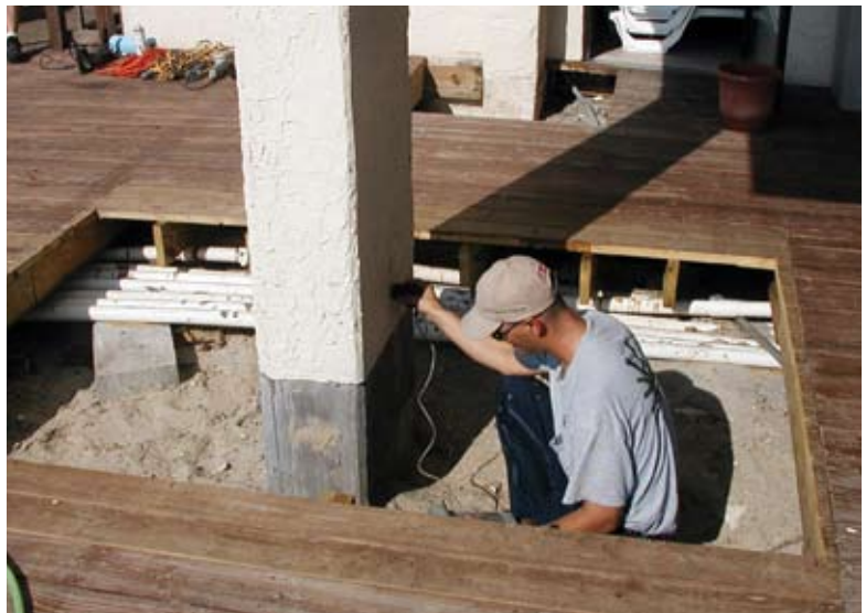
Locating reinforcing steel prior to galvanic anode installation
