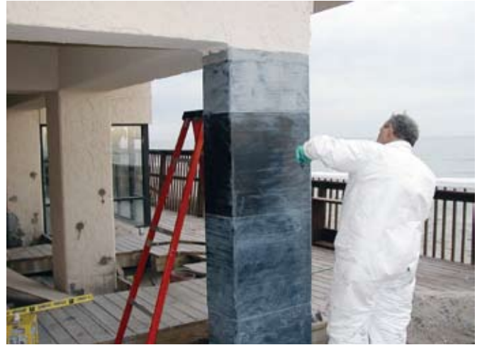
Installation of carbon-fiber strengthening system
