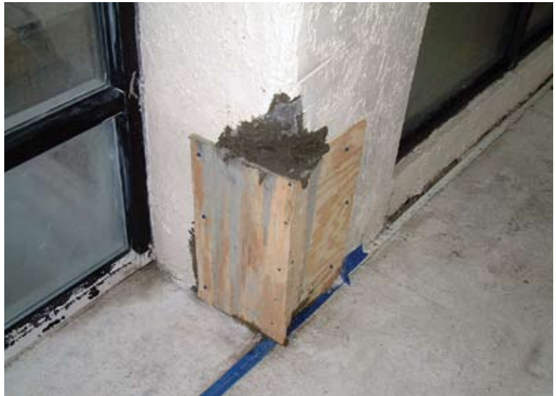
Concrete patch repair
