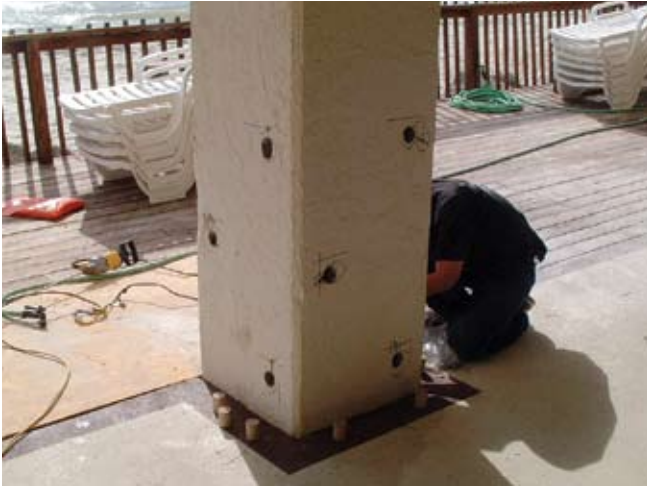
Holes drilled prior to anode installation
