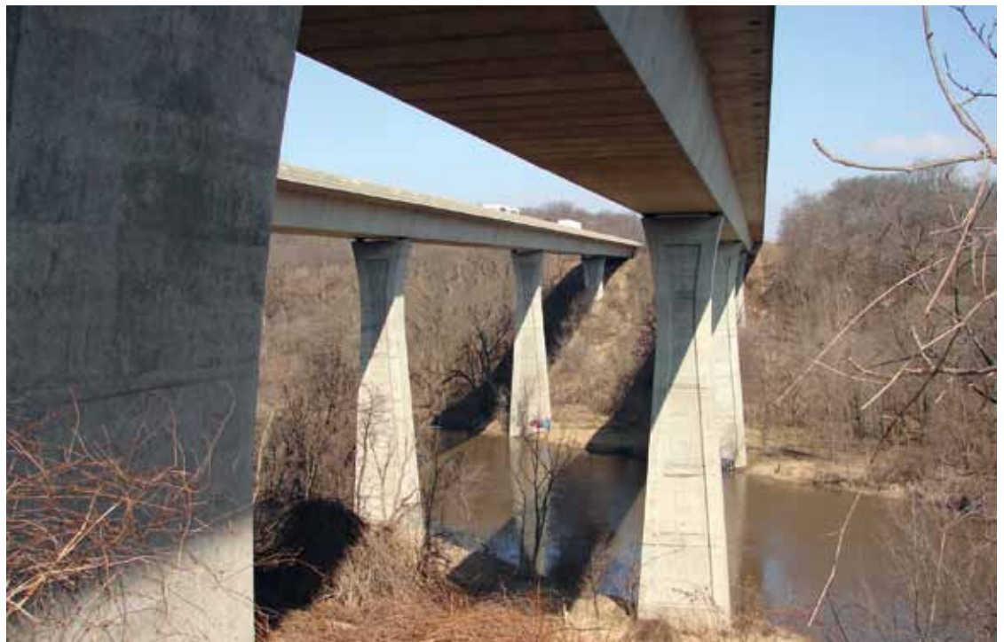
The Kishwaukee River Bridge
