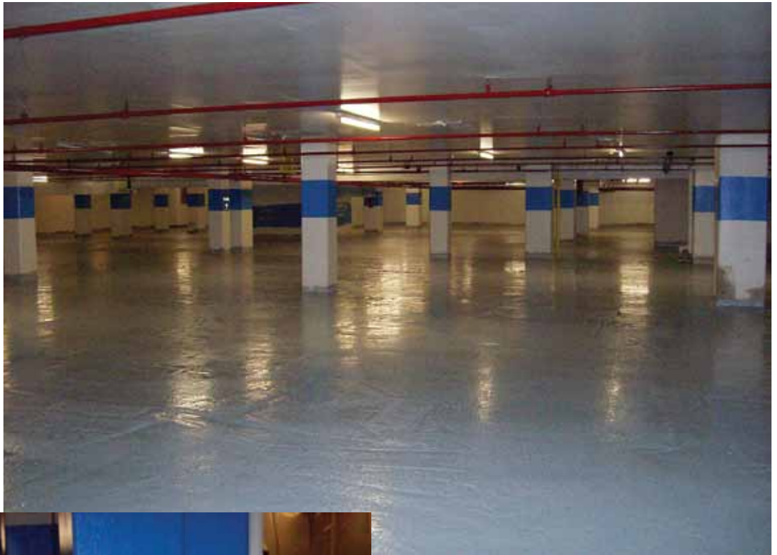
Installed base coat
