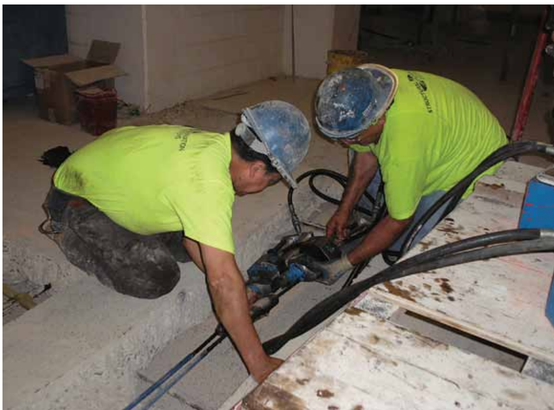
Stressing of post-tensioning cables
