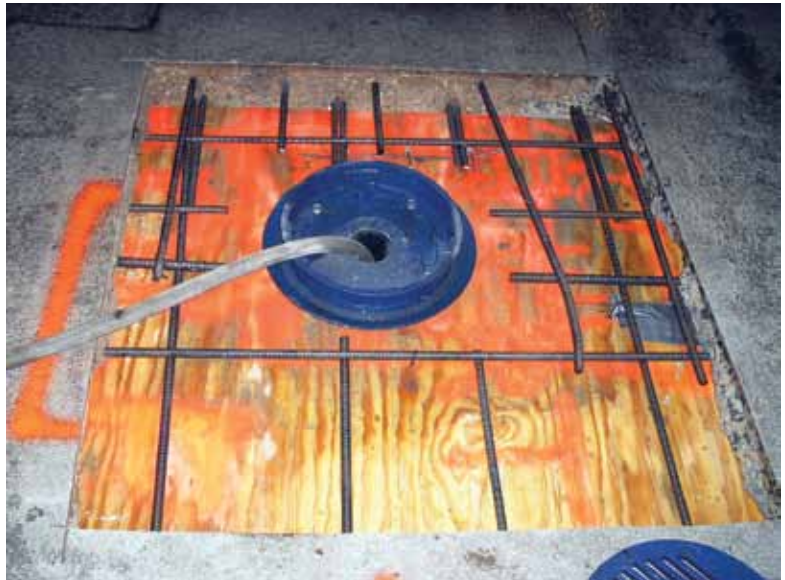
Full-depth hole for new drain installation
