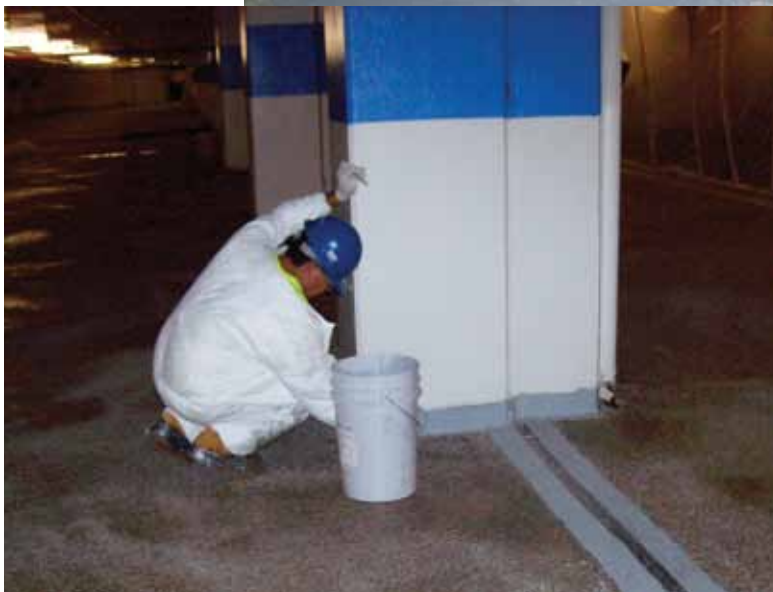
Installing coating detail on column
