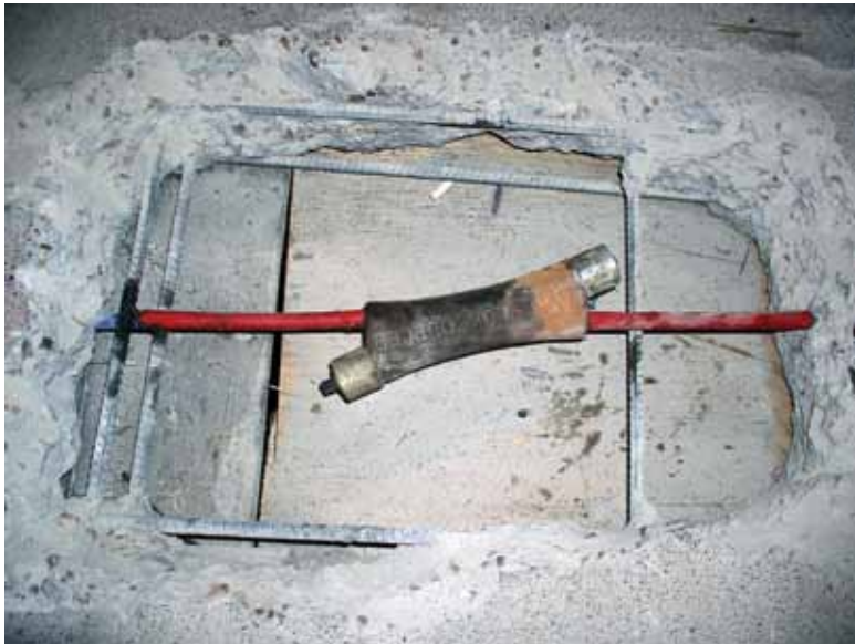
Fig. 7: Center stressing splice for monostrand system
