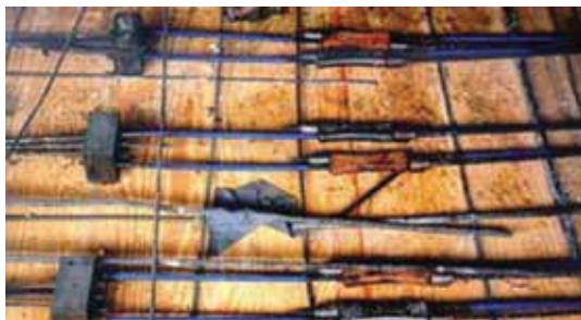
Fig. 8: Monostrand to wire system splice (after VanOcker [2005])
