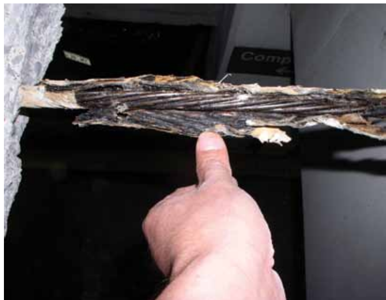
Fig. 4: Emulsified PT coating (grease) from a paper-wrapped system
