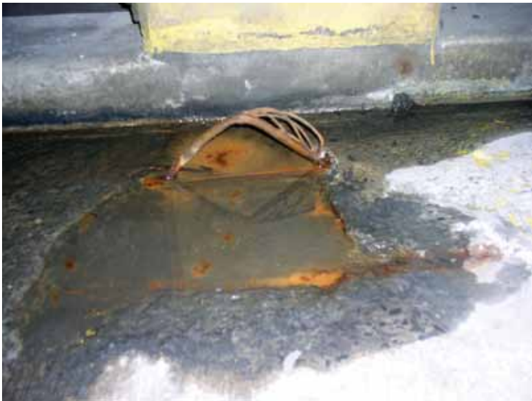
Fig. 6: Post-tensioning tendon failure due to corrosion
