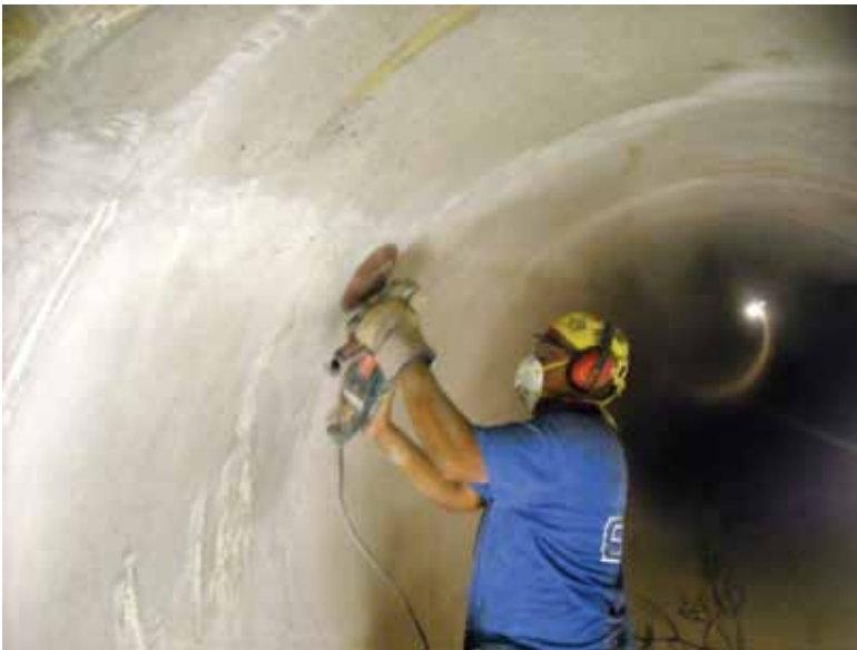
Fig. 4: Preparation work prior to installation of FRP lining
