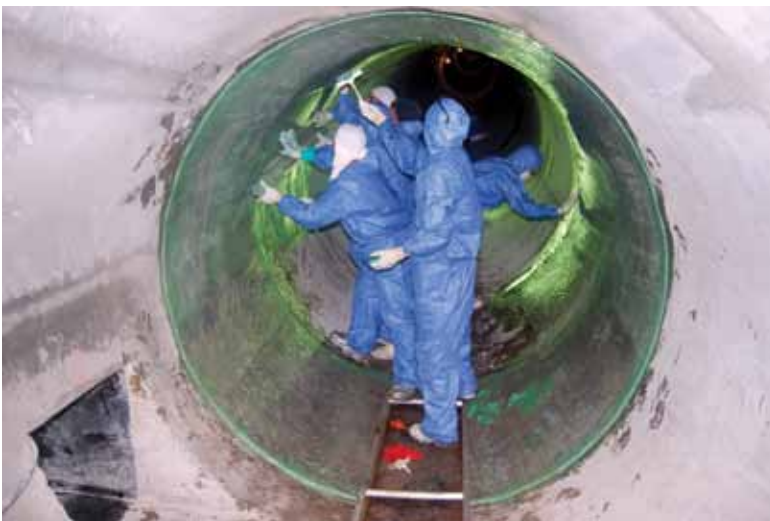
Fig. 5: Installation of FRP sheets on the interior surface of the pipeline
