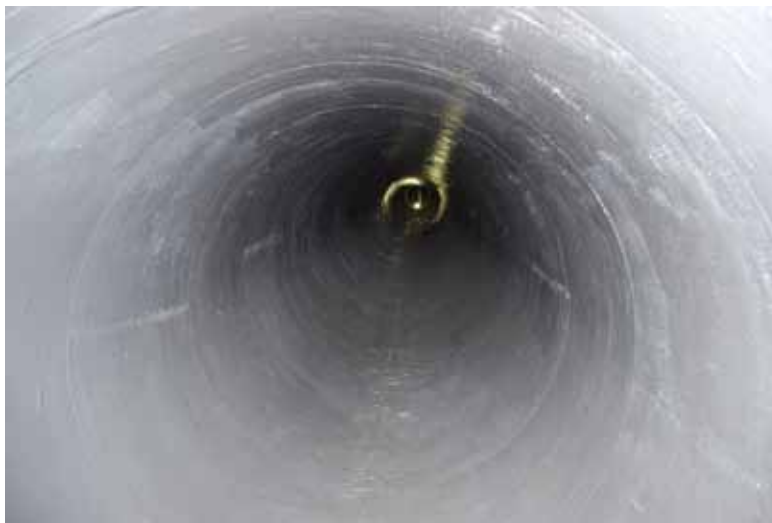
Fig. 6: Completed segment of pipeline prior to testing
