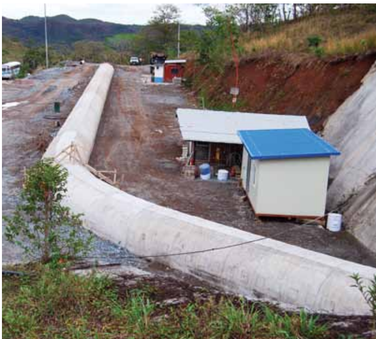
Fig. 1: Aboveground segment of the El Encanto pipeline
