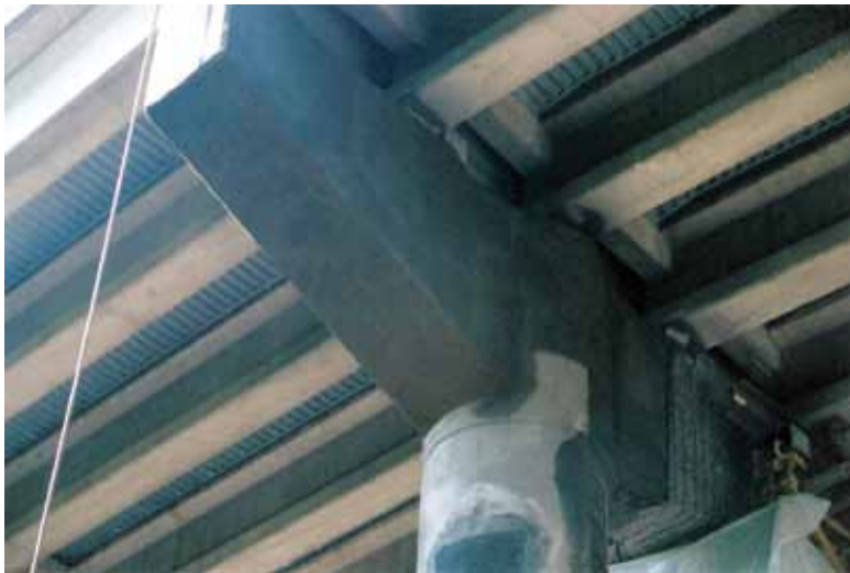
After shot of repair on bridge
