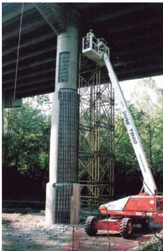
Bridge support ready for repair material
