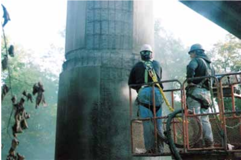
Shotcrete being applied to Noblestown Road Bridge
