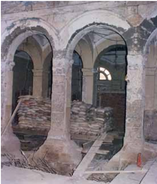
Load test on single pile. Foundation of existing granite columns also shown
