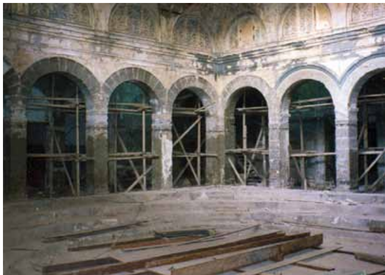
Main Hall at the beginning of work
