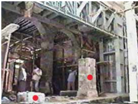
Truss frames after removing the two granite columns, indicated by a dot (●)
