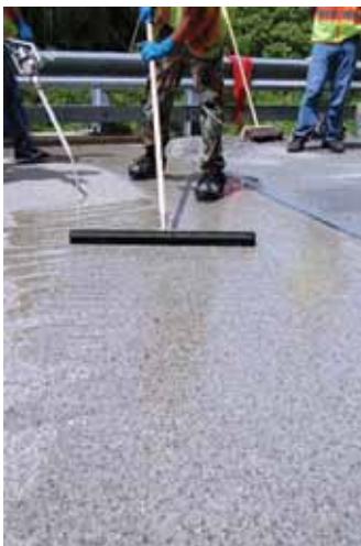
Fig. 4: Spreading epoxy with a notched squeegee
