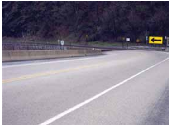
Fig. 8(b): Completed TPCO
