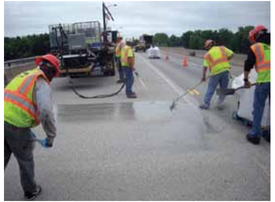
Fig. 6: Applying the second lift of TPCO
