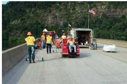
Fig. 2: Ride-on shotblast machine. The magnet bar on wheels to the left is collecting excess metal shot
