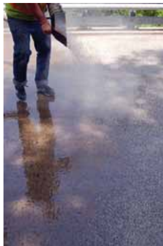
Fig. 5: Applying flint rock by aggregate blower
