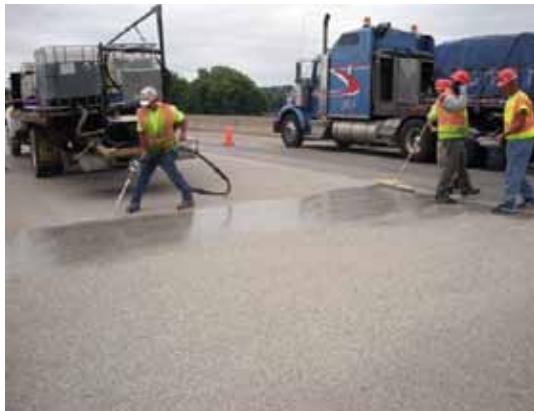
Fig. 3: Plural pump dispensing proper ratio of epoxy Parts A and B
