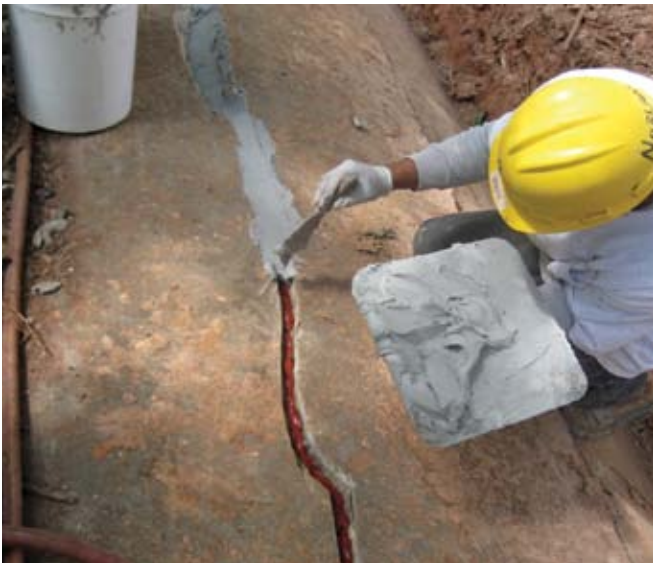
Fig. 6: Swellable water stop capped with an epoxy
