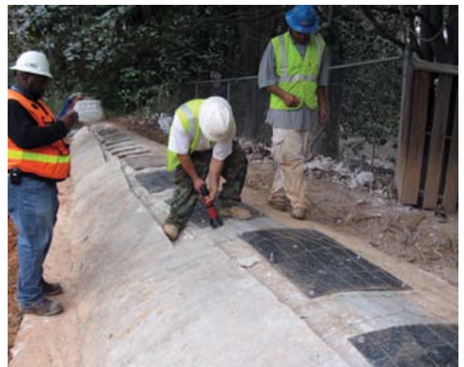
Fig. 2: Use of steel plates followed by placement of fresh concrete
