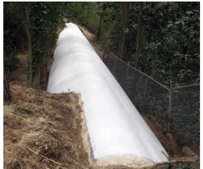
Fig. 10: The repaired pipe after being coated with a water-based acrylic coating
