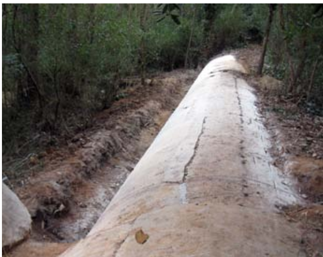
Fig. 1: Ninety in. (2290 mm) sewer pipe located in Atlanta, GA
