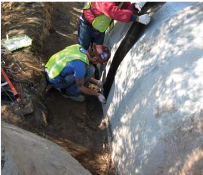
Fig. 7: Dry layup technique used to install the fabric
