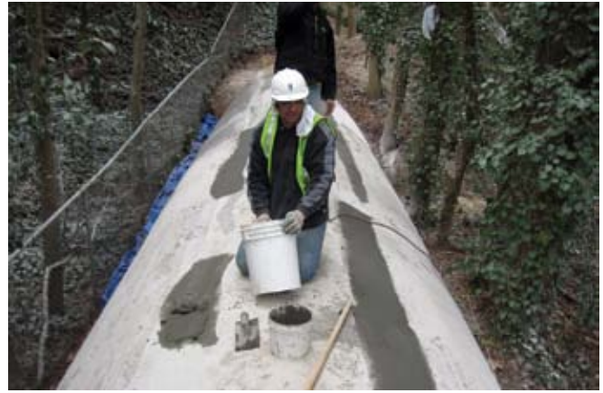
Fig. 4: Application of the repair material
