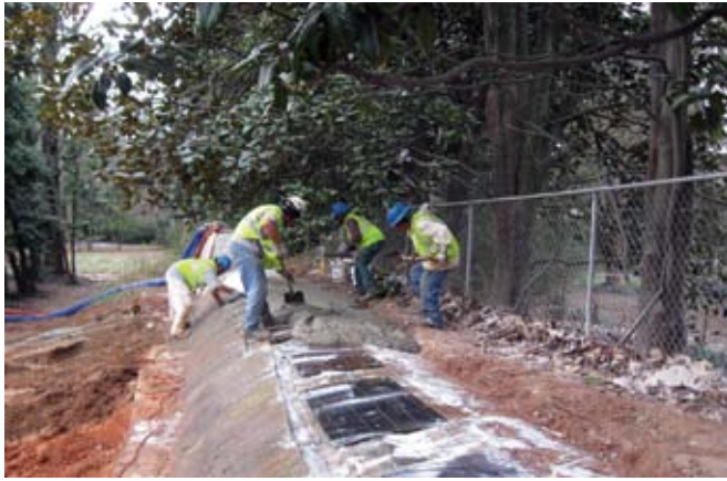
Fig. 3: Steel mesh was added prior to the concrete placement
