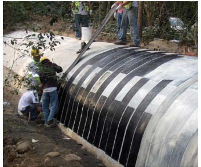
Fig. 8: Multiple layers of CFRP installed
